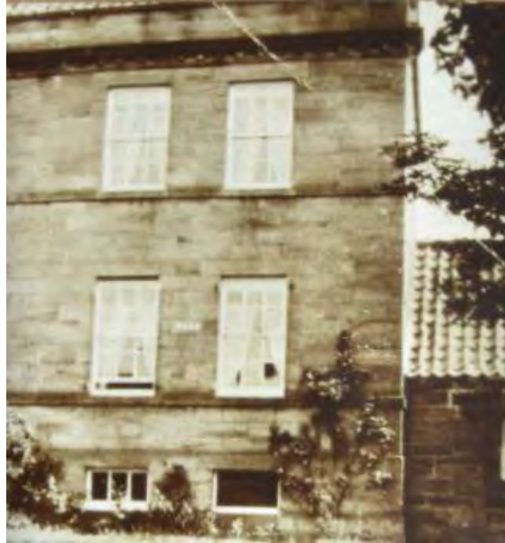
Figure 7: Front elevation right side - note six over six sash windows still in place - Source: Elvington Park Limited
