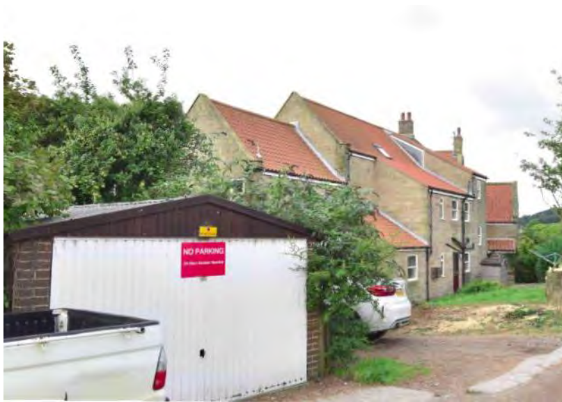
Figure 13: Rear elevation looking South-West - Source: Elvington Park Limited
