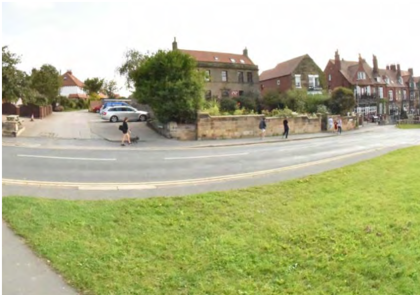
Figure 17: View across road towards The Bay Tree looking East - Note how trees shield side elevation from view - Source: Elvington Park Limited
