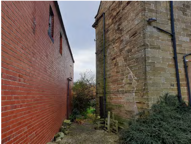
Figure 11: Southern end of original building with ghost of smaller structure now removed. Note the red brick of the neighbouring structure. – Source: Author
