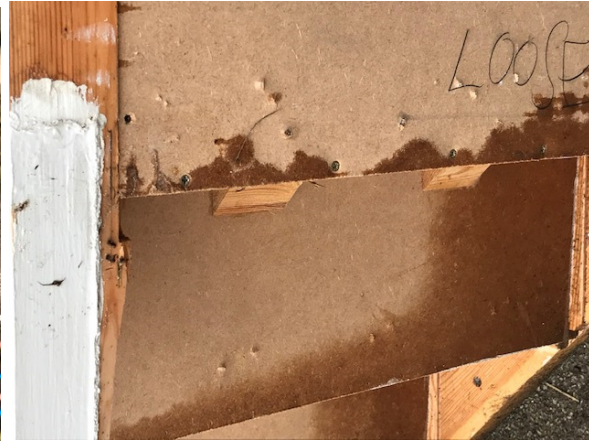
MDF stair removed
