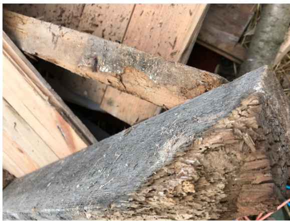
Rotten timber floor removed
