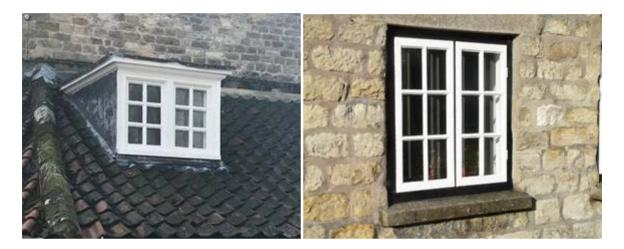
All replacement windows should be of traditional construction incorporating weight bearing glazing bars. The use of slim d/g units will be necessary in order to achieve this and should be of 4:4:4 or 4:6:4 profile as a maximum. While the sectional details can be conditioned as part of an approval, we will require confirmation of this approach and amended plans prior to determination.
