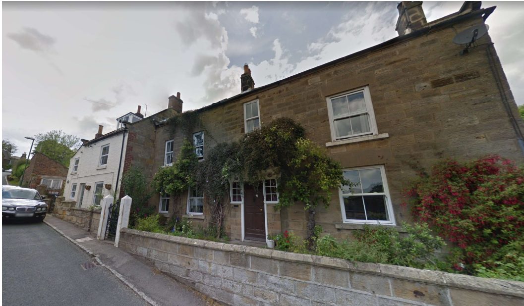
Grove Cottage (with Stone Gable End) & Neighbouring Property
