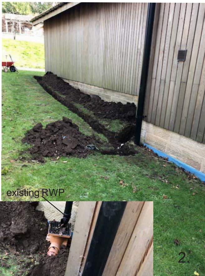
west elevation from south showing excavations to expose existing drains
