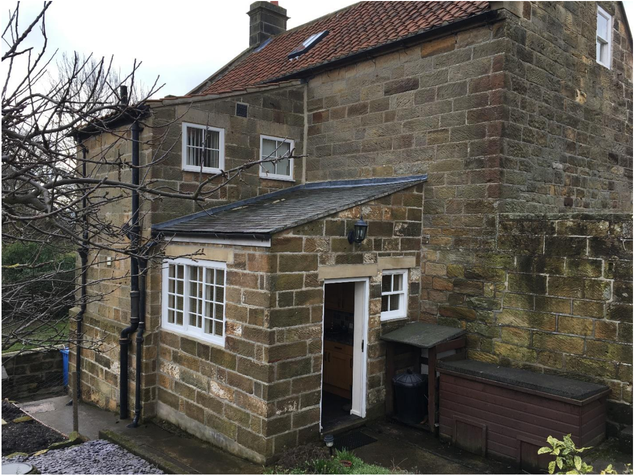
Photograph 1 Rear Elevation showing Mono Pitch Extensions
