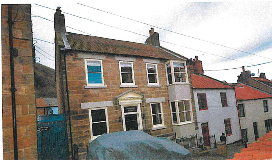
East – Front elevations of Balmoral House onto Church Street.
