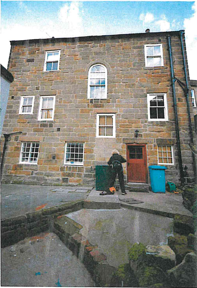
Rear – West Elevation onto private yard.
