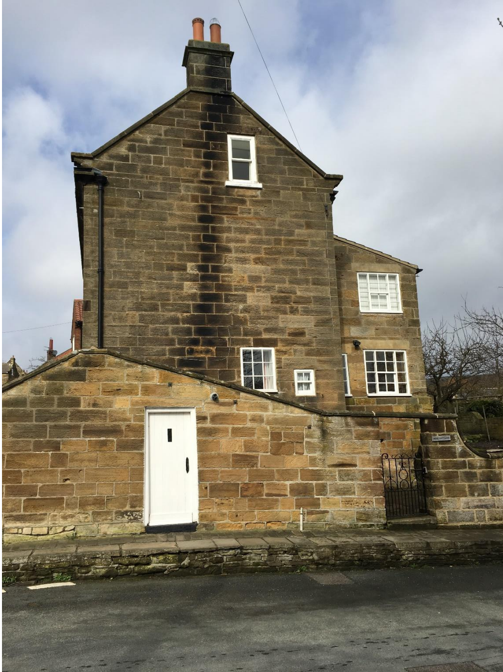
Photograph 3 Side Elevation (East)
