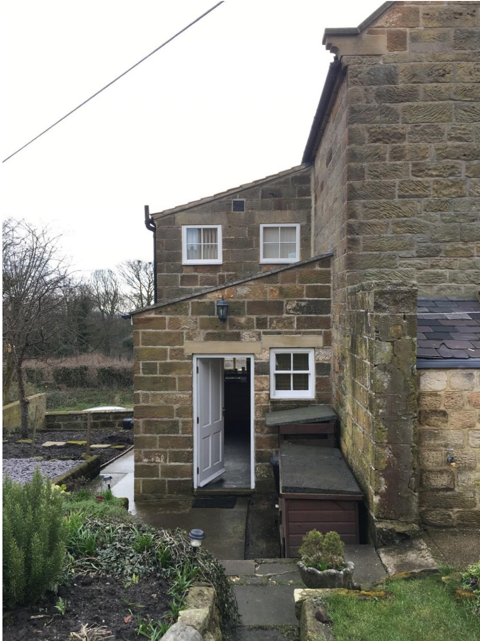
Photograph 2 Rear/West Side View
