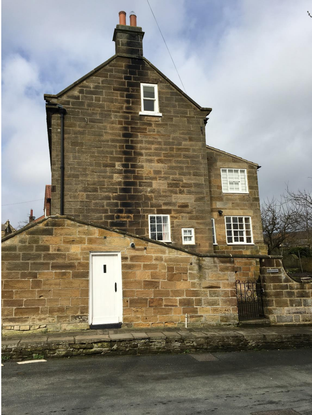
Photograph 3 Side Elevation (East)
