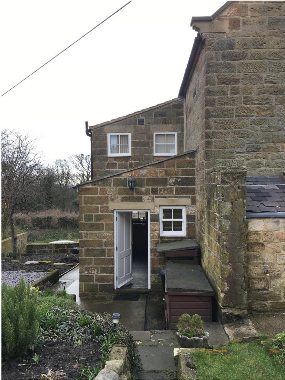
Photograph 2 Rear/West Side View
