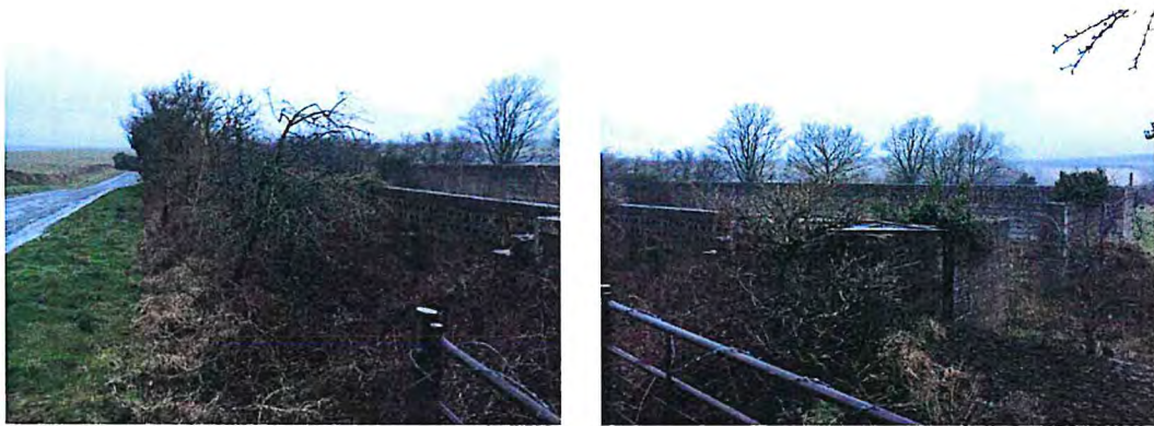
Photograph 1: Representative views of southern boundary section – northern site (left) and view over concrete structure (right).
