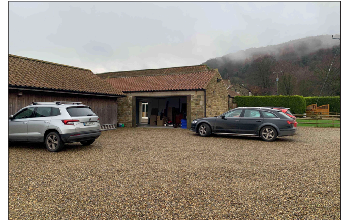
Garage and rear of stables
