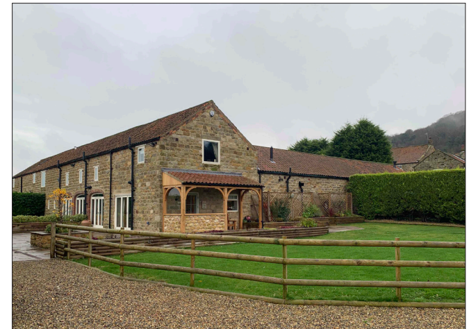
North east corner of barns
