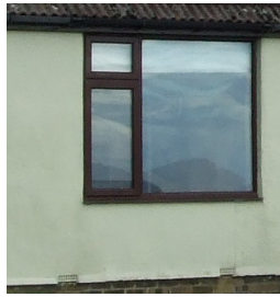
PVCu Framed Windows to dwelling
