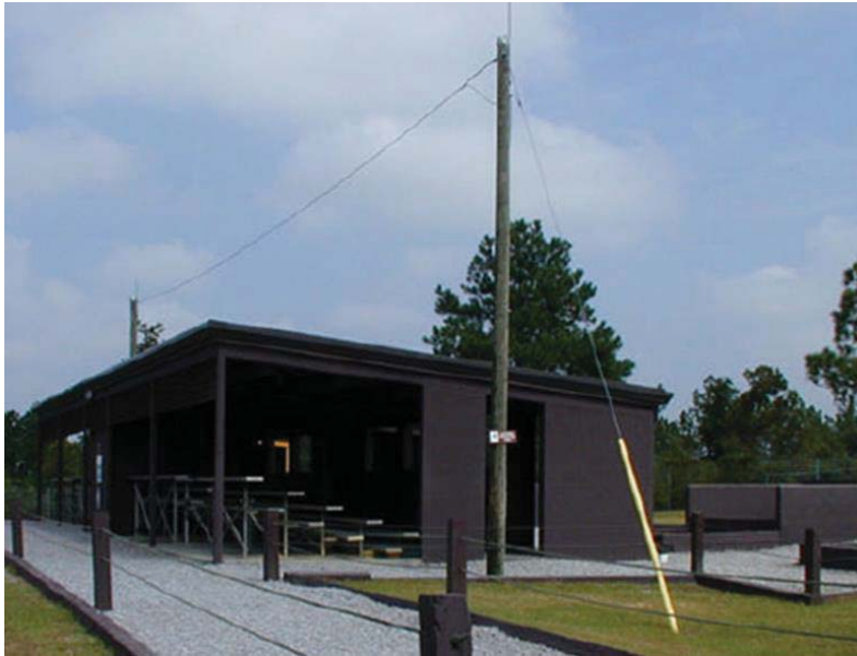
Figure 21: Example of lightning protection over a shed
