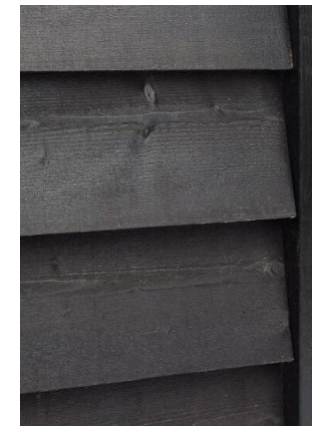
horizontal shiplap boarding to have black stain
