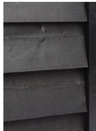
horizontal shiplap boarding to have black stain
