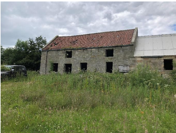
Plate 17 South aspect of Building 4
