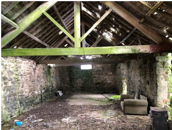
Plate 27 Interior of Building 6
