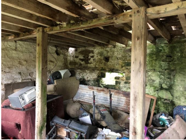
Plate 19 Interior of Building 4
