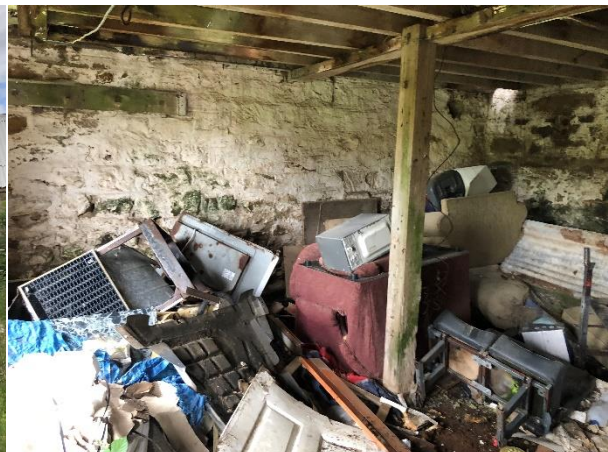
Plate 18 Interior of Building 4
