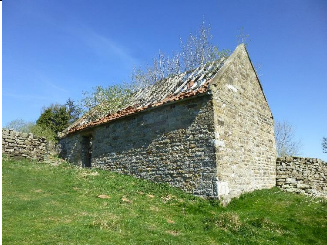
Barn Group Two West Elevation
