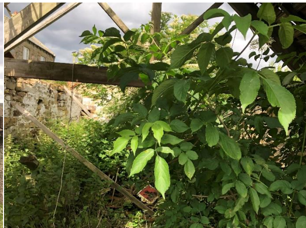
Plate 12 Interior of Building 2
