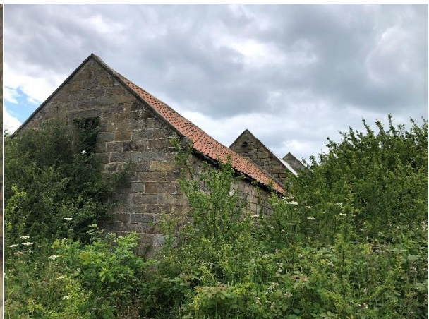
Plate 24 North aspect of Building 6
