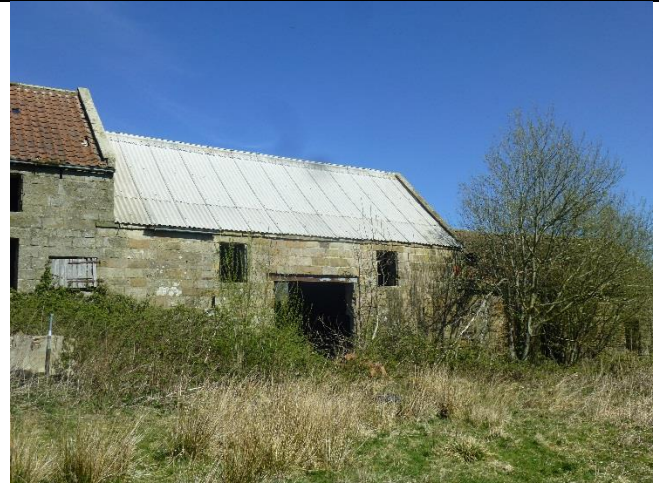
Barn Group One South Elevation
