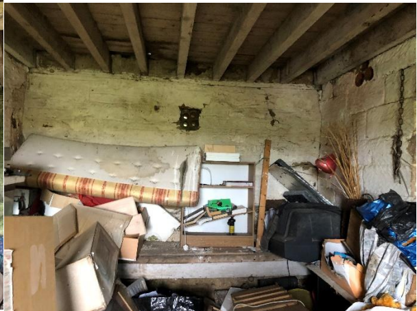
Plate 20 Interior of Building 4
