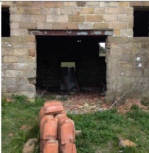
Steel Lintel on Barn Group One
