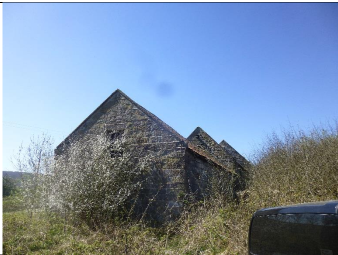
Barn Group One East Elevation
