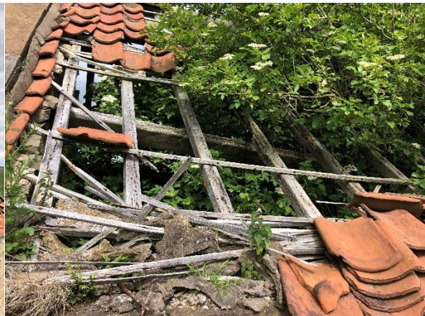
Plate 16 Detail of Building 3
