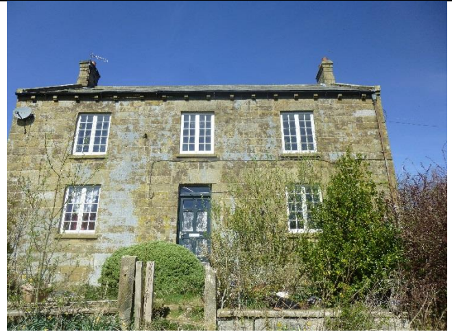
Farmhouse South Elevation
