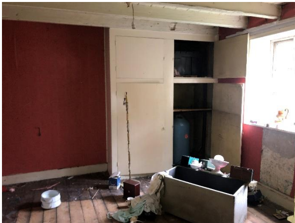
Plate 5 Interior lower floors of Building 1
