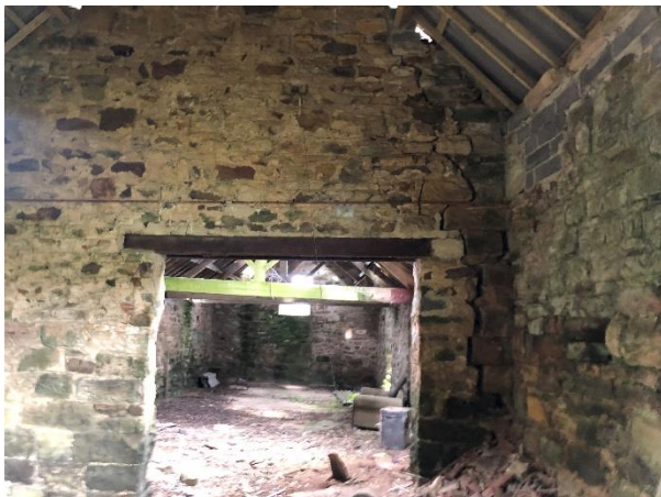
Plate 23 Interior of Building 5 and 6
