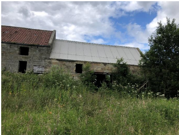
Plate 21 South aspect of Building 5
