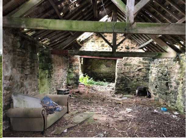
Plate 26 Interior of Building 6
