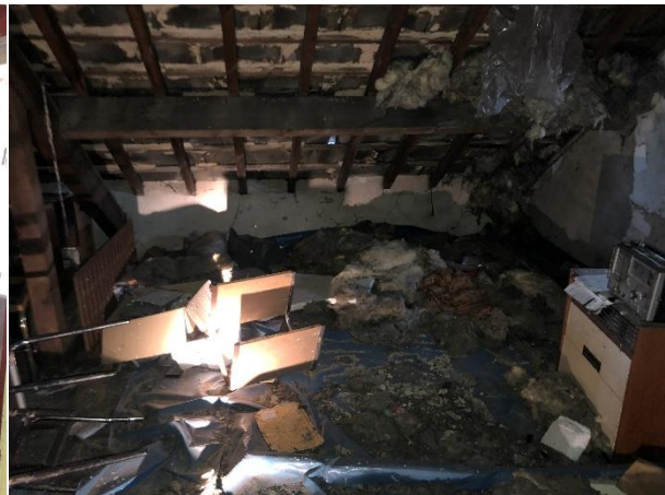
Plate 6 Attic of Building 1
