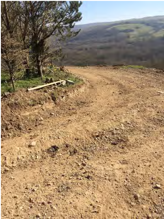
Fig 5. – view to north from 1st T junction.
