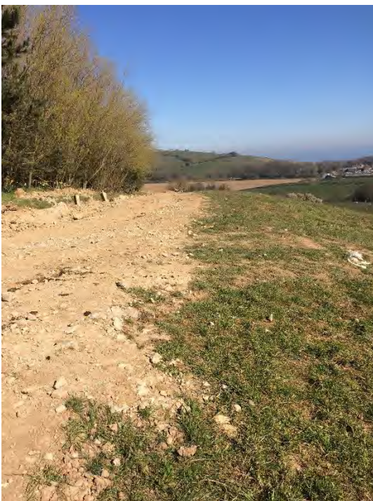
Fig 7. - 2nd T junction proceeding along previously shored up edge.
