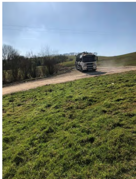
Fig 16. – Tanker accessing site and septic tank.
