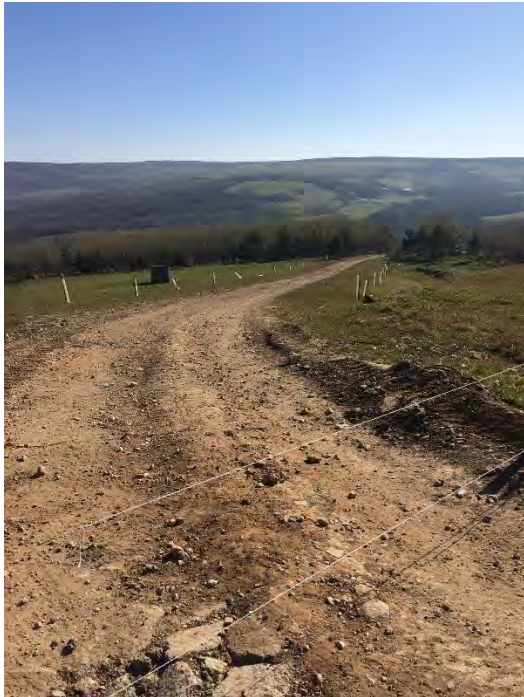
Fig 1. - From electric gate looking down hill.
