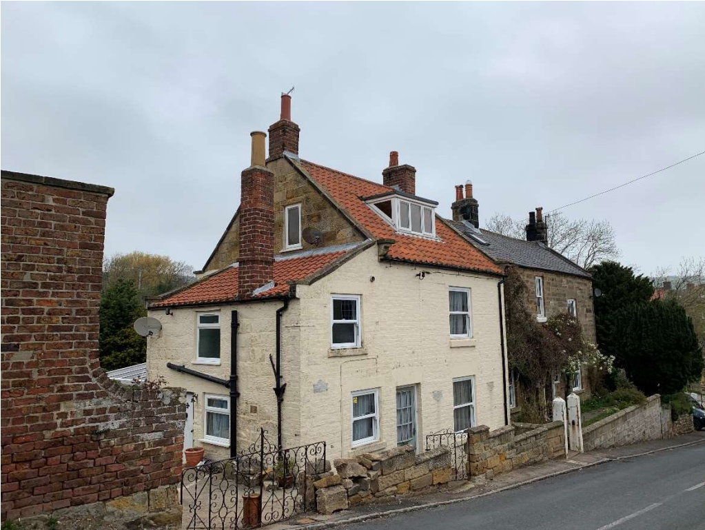
Photograph 3 - Existing Gated Access & Main Property
