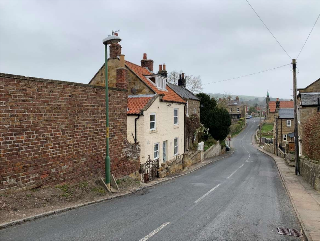
Photograph 4 - Existing Gated Access & Outbuilding Wall (to be demolished)
