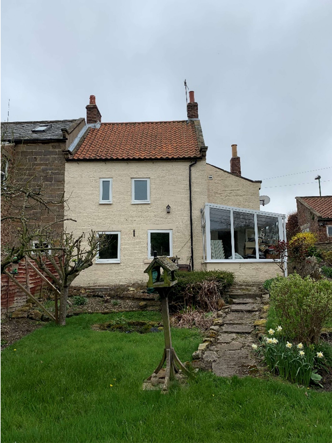
Photograph 2 - Existing Rear Elevation
