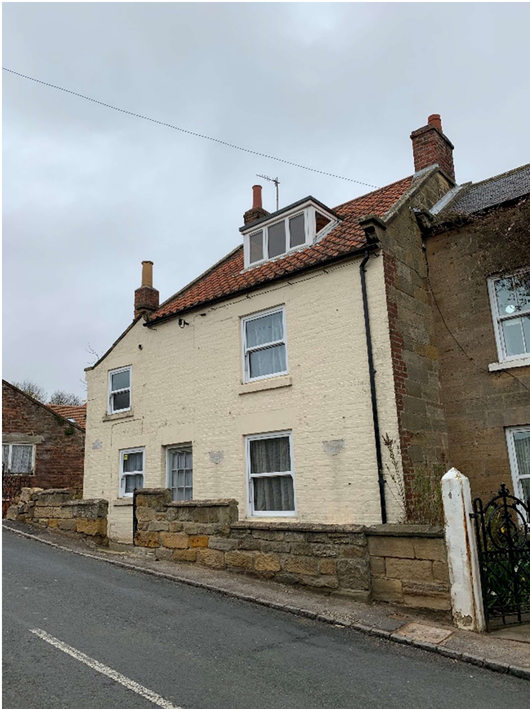
Photograph 1 - Existing Front Elevation
