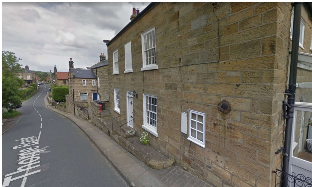
Photograph 6 – Example of stone built properties directly opposite appeal site.
