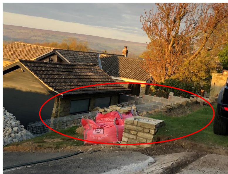
2 no. photos from rear facing Egton Road.
