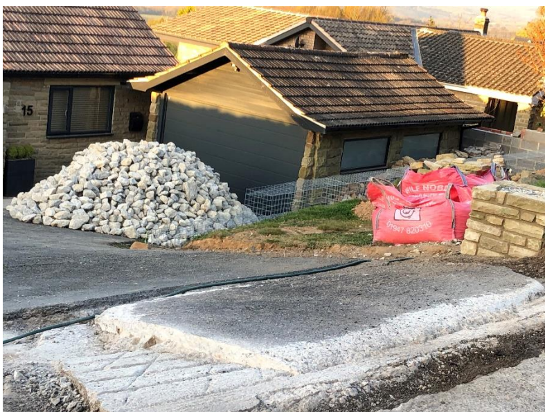
Example 4 - No 15 New off street parking area and retaining walls.
