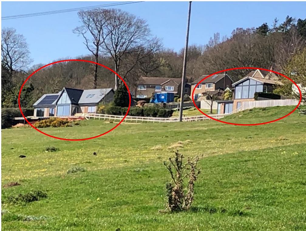
Example 3 - Nos 17 and 21 Egton Road, Aislaby. Photo from rear facing south to Eskdaleside.
