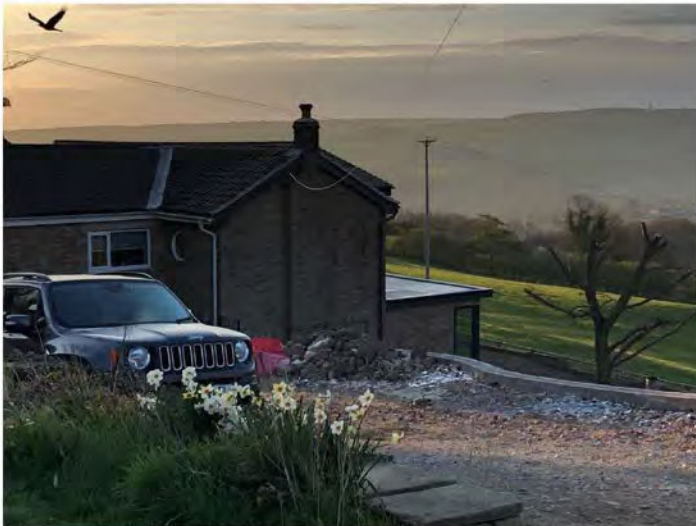
Example 3 – No. 17 Extension and new access drive. Photo from rear facing Egton Road.
