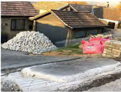
Example 4 - No 15 New off street parking area and retaining walls.
