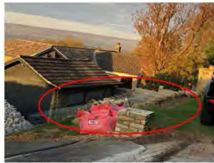
2 no. photos from rear facing Egton Road.
