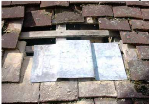
Plate 10 - Diagrams of a lead bat tile
