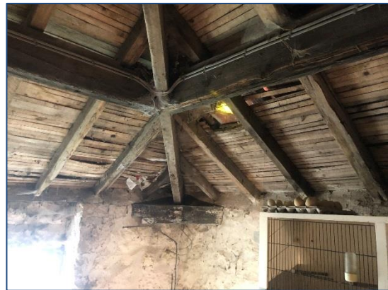
Photo 2: Internal view of lath lined roof of Building 1
