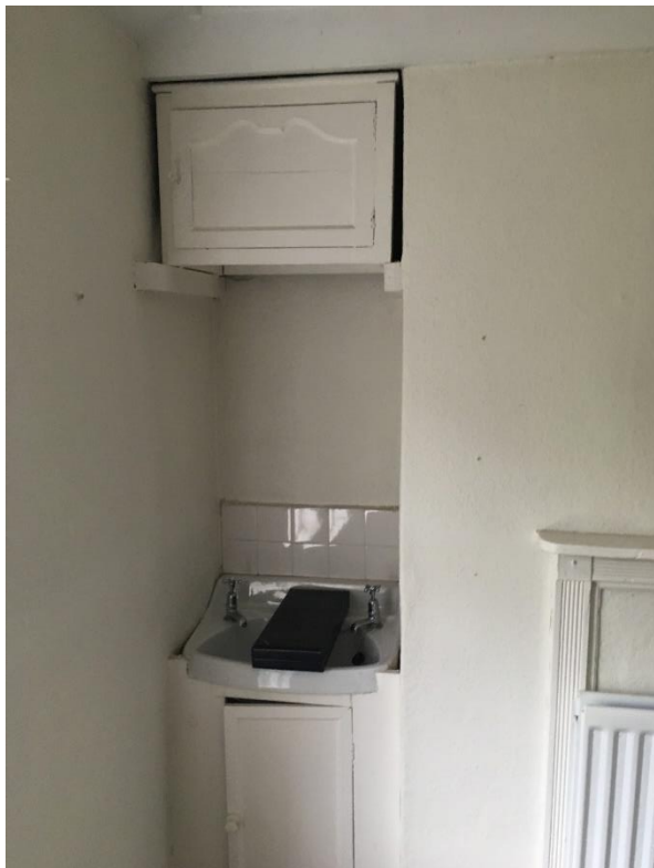
Fig 39. - Second floor rear bedroom – sink and cupboard in alcove
