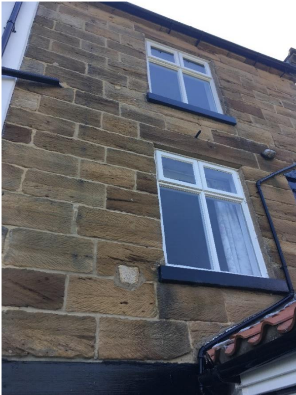
Fig 8. – Rear elevation first and second floor windows and stonework
