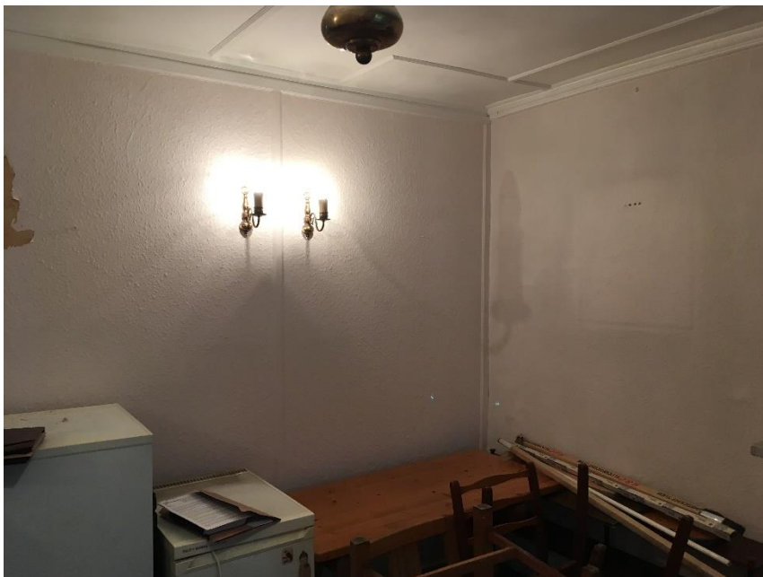
Fig 18. – Ground floor lounge – stoothing wall and panel ceiling
