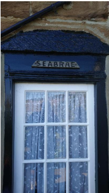
Fig 9. – Rear lower ground floor door
