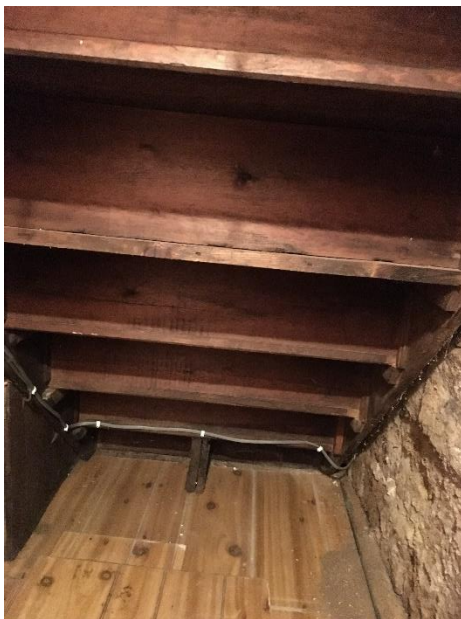
Fig 22. – Under stairs cupboard off kitchen
