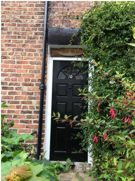
Fig 6. – Sea Brae, Robin Hoods Bay - traditional front door and boxed in fan light
