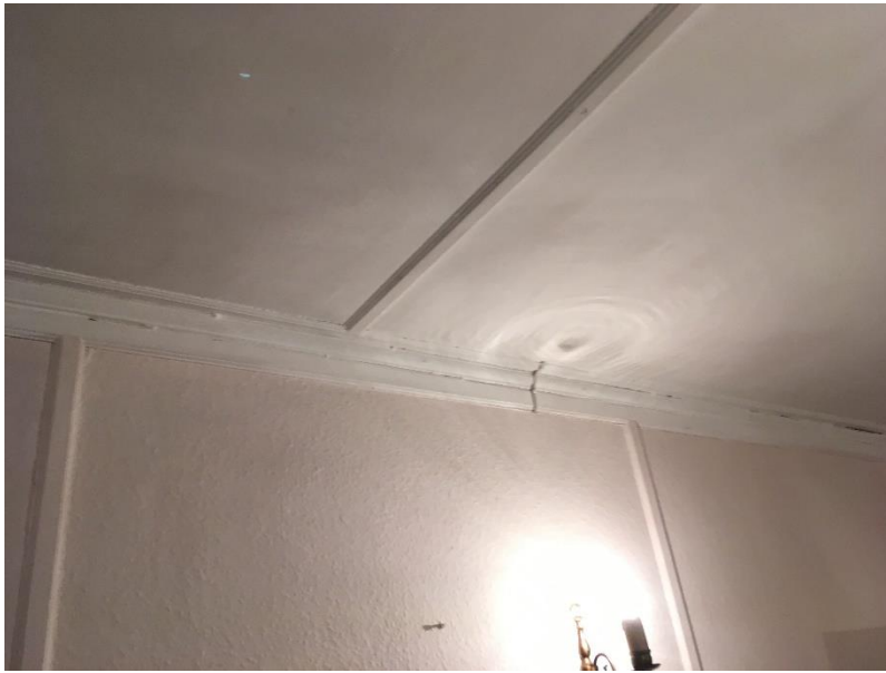
Fig 19. – Ground floor lounge - non traditional wall and ceiling panelling
