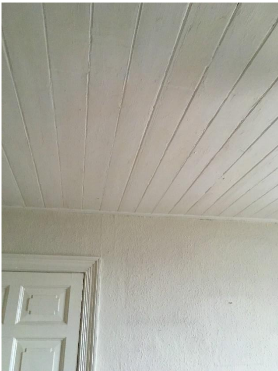
Fig 30. – First floor sitting room – traditionally boarded ceiling
