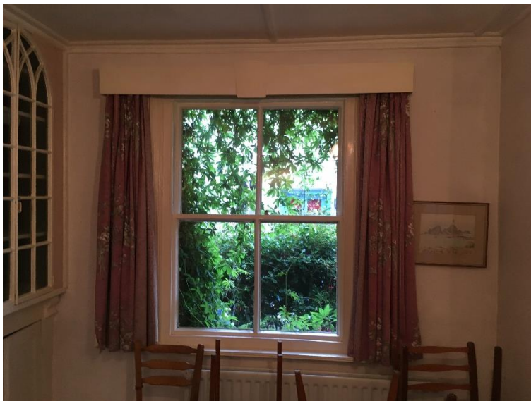
Fig 13. – Ground floor lounge – principle elevation window
