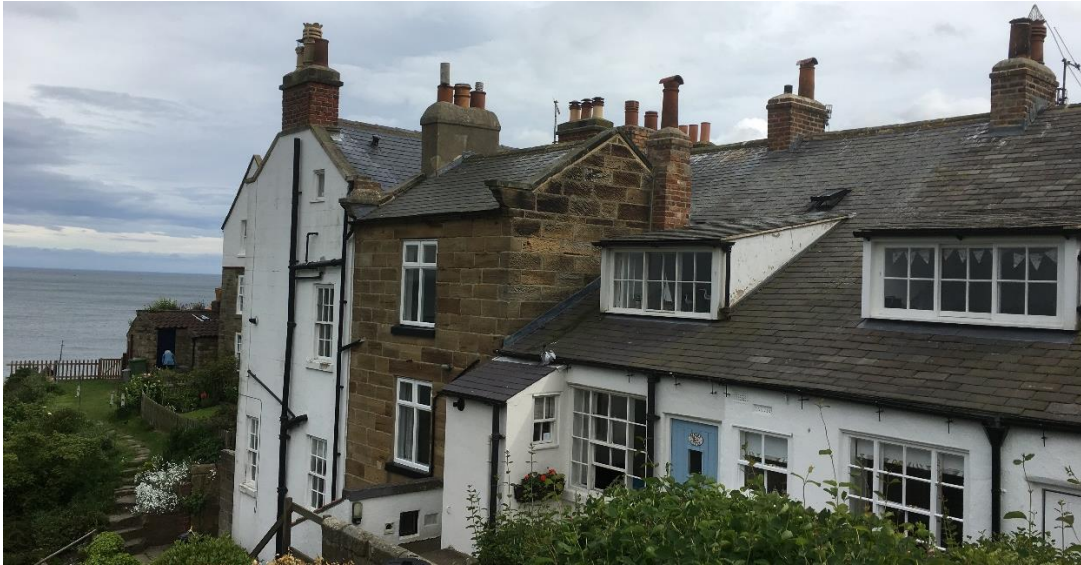
Fig 8. – Rear elevation of The Esplanade including Sea View and High Sea View.
