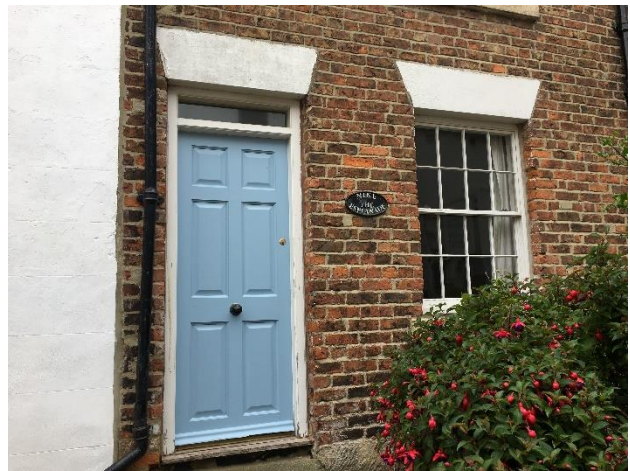
Fig 4. – Door serving No. 8 The Esplanade – style and appearance to be replicated at Sea Brae.
