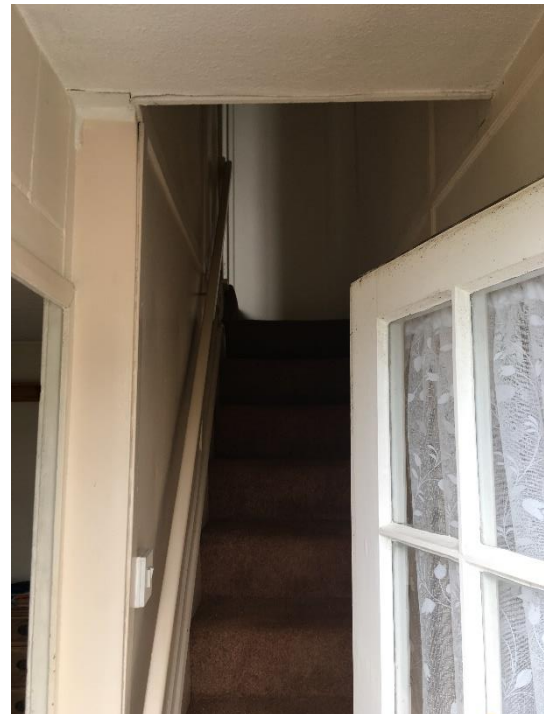
Fig 35. – First floor rear staircase
