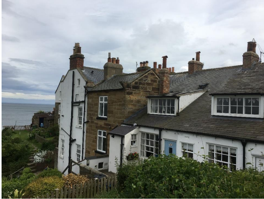
Fig 1. – Sea Brae, 10 The Esplanade, Robin Hoods Bay – stone and slate property in centre
