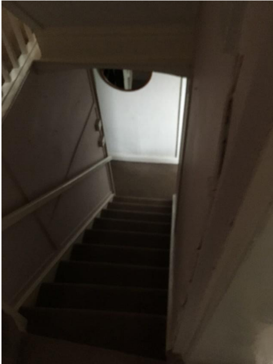
Fig 23. – Looking down first floor staircase
