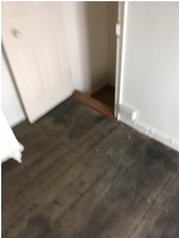
Fig 29. – First floor sitting room and traditional floorboards
