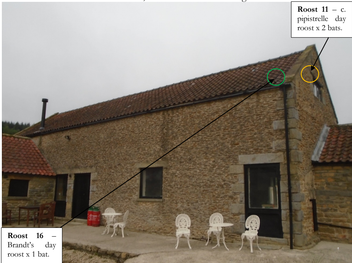
Plate 5 – barn, south elevation and east gable.
