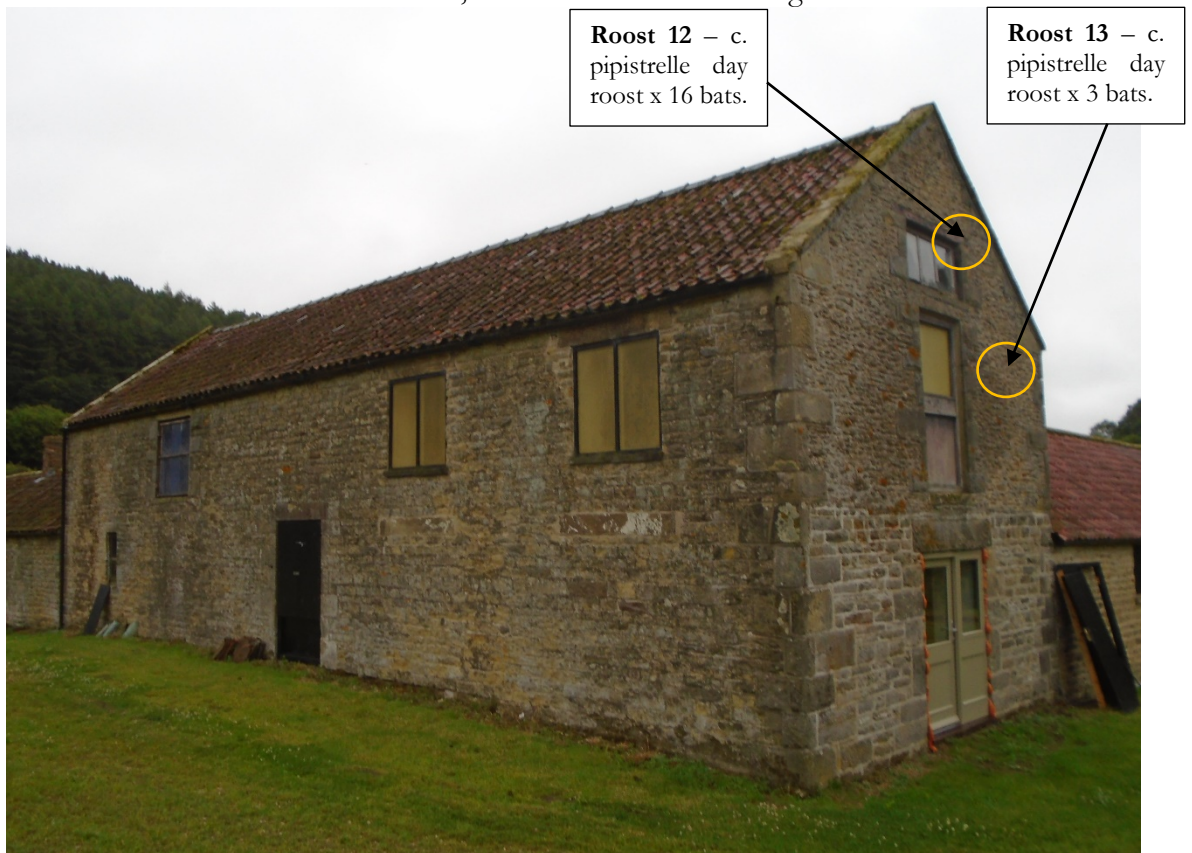
Plate 6 – barn, north elevation and west gable.
