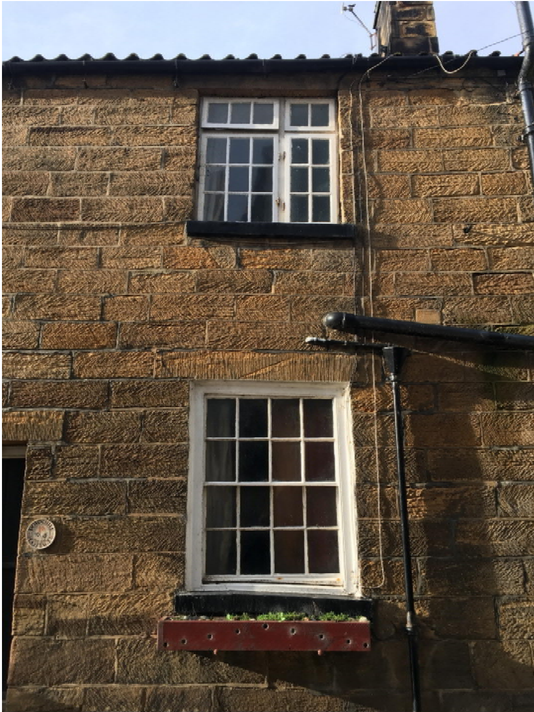
Photograph 6 Part Front Elevation, W2 and W4
