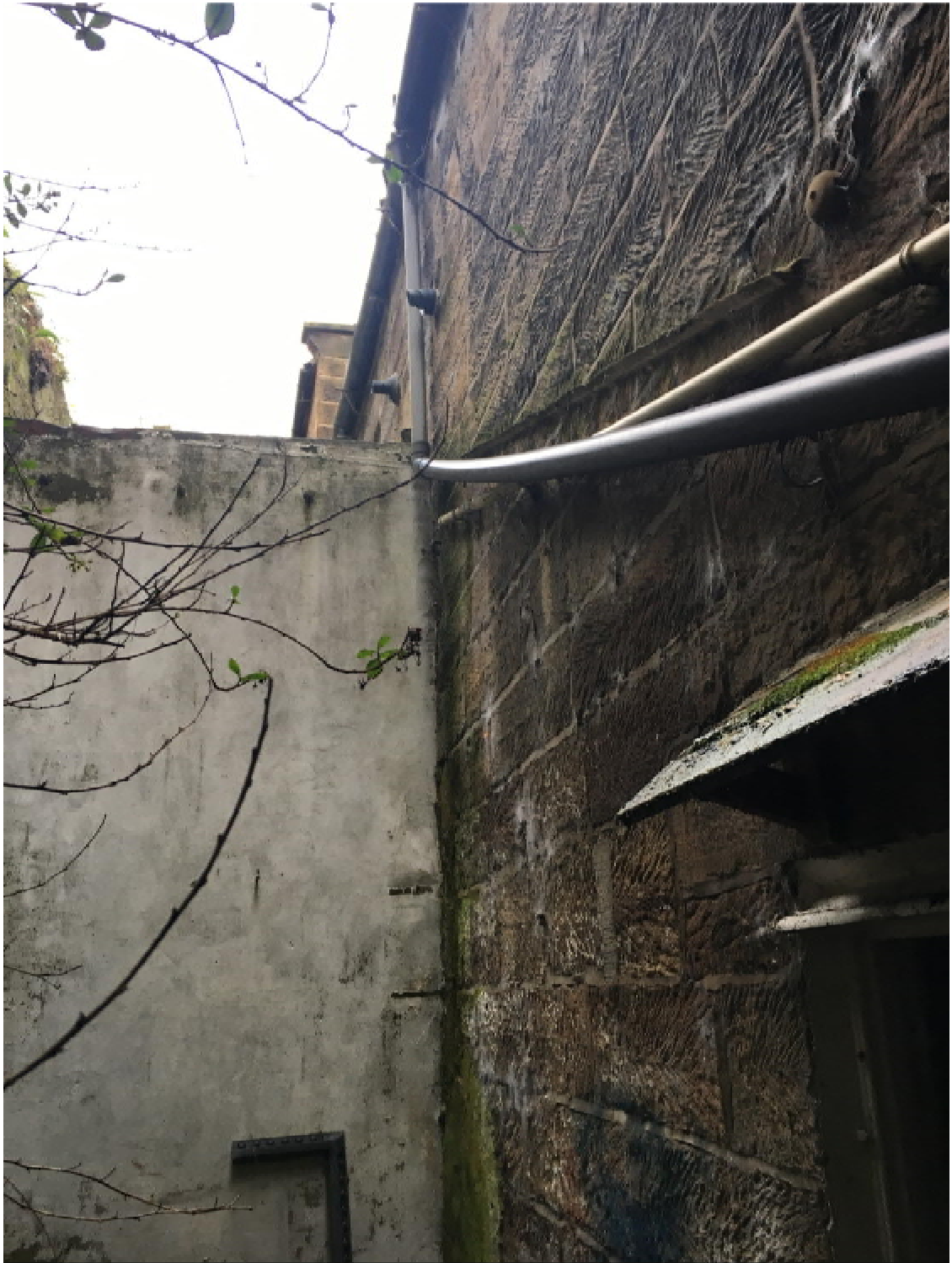
Photograph 8 Rear Yard looking at Party Wall of Beadle Cottage
