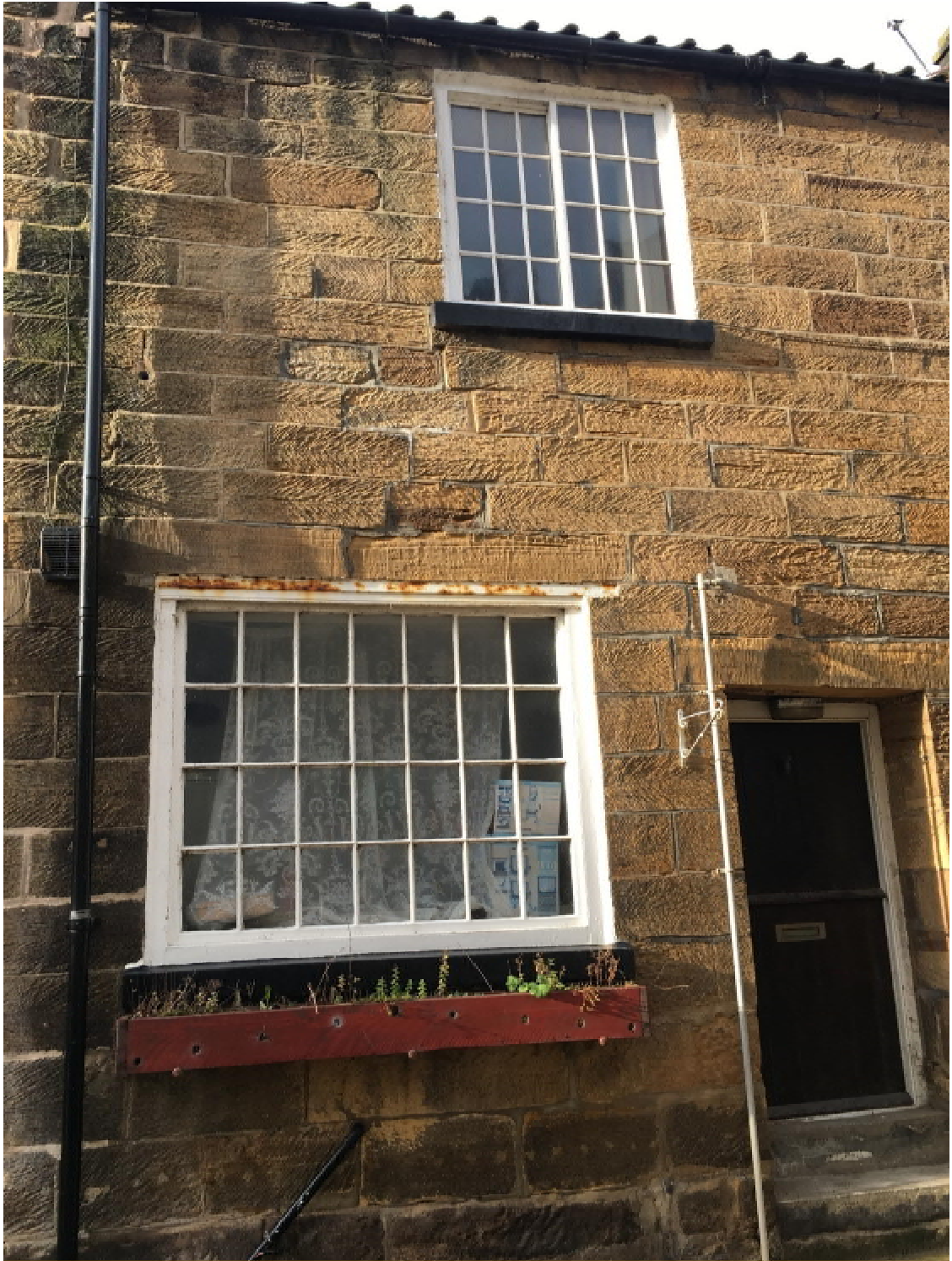
Photograph 5 Part Front Elevation, W1 and W3
