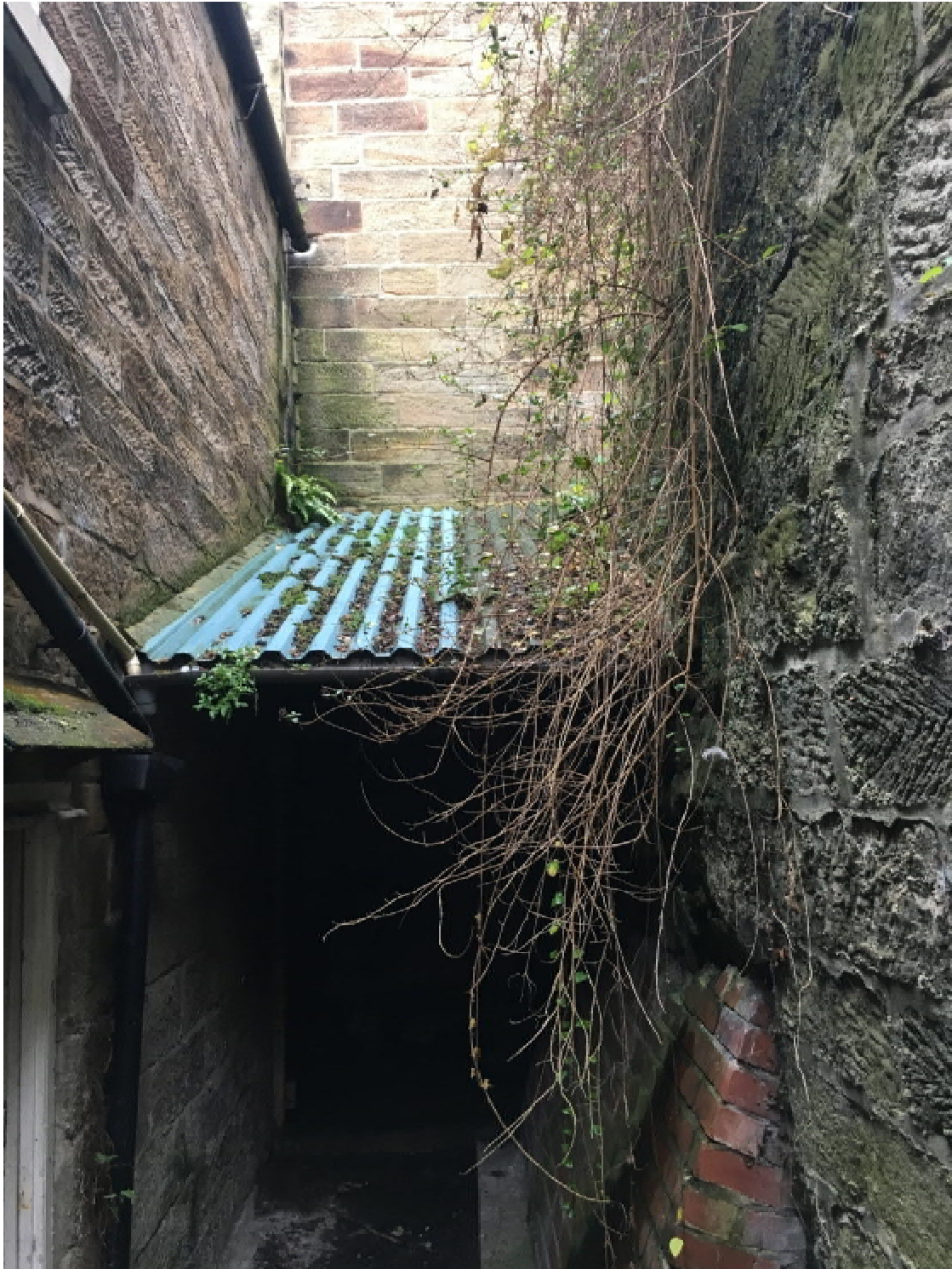
Photograph 9 Rear Yard looking at Party Wall to the south Note; covered area and brick buttress
