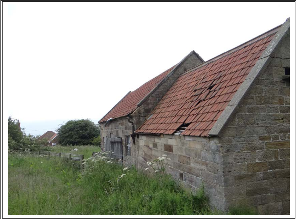
Photo 3 East elevations of Graystone Barn
