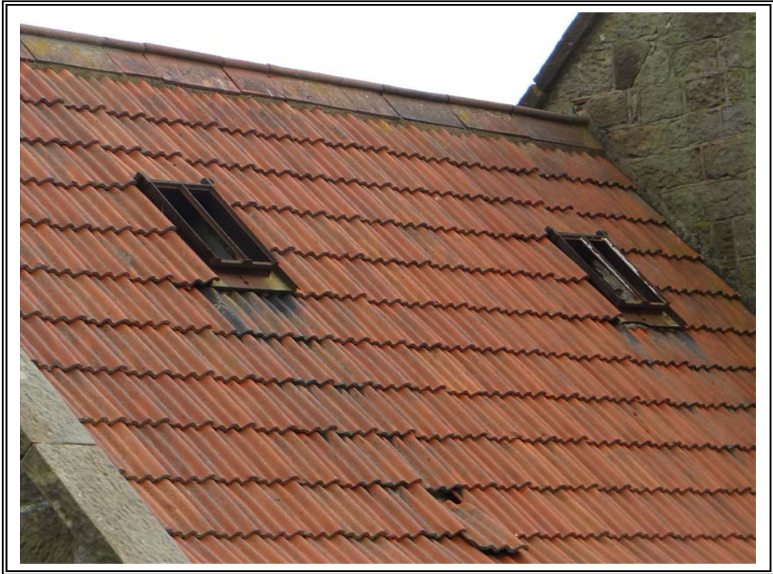
Photo 4 Existing rooflights to one of the roof slopes of Graystone Barn.
