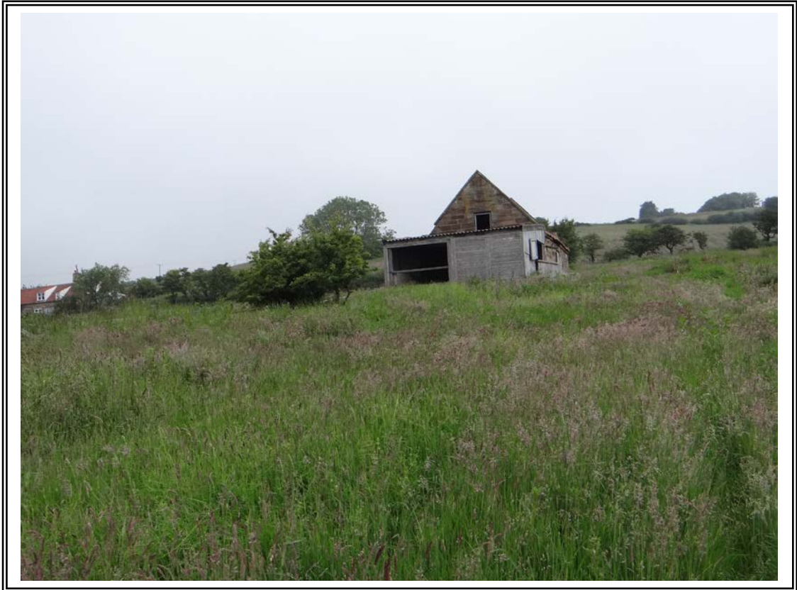
Photo 6 South gable and timber framed lean to of Barn B
