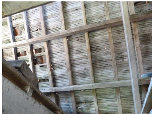
Photo 4 Wooden lath lining and wood floor
