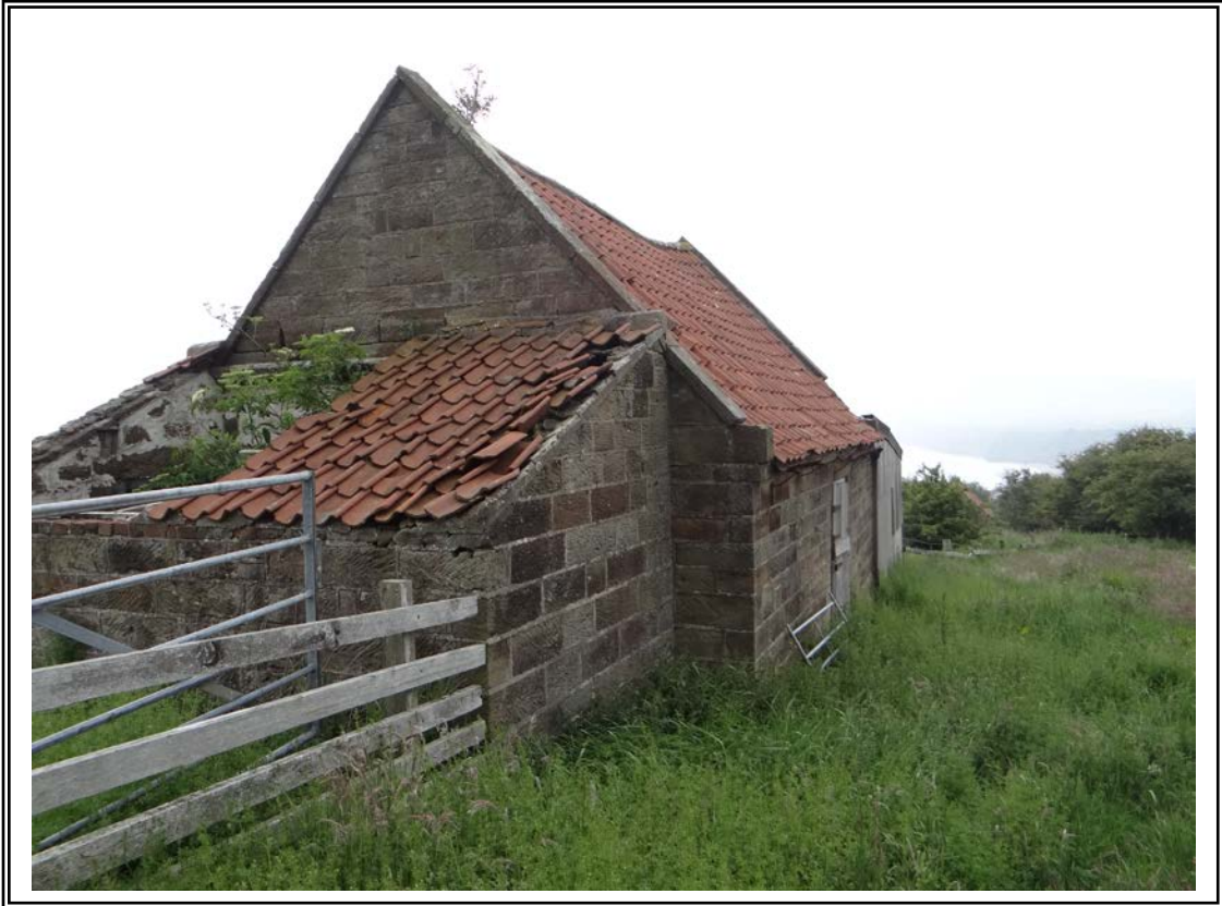
Photo 7 West elevation of Barn B.
