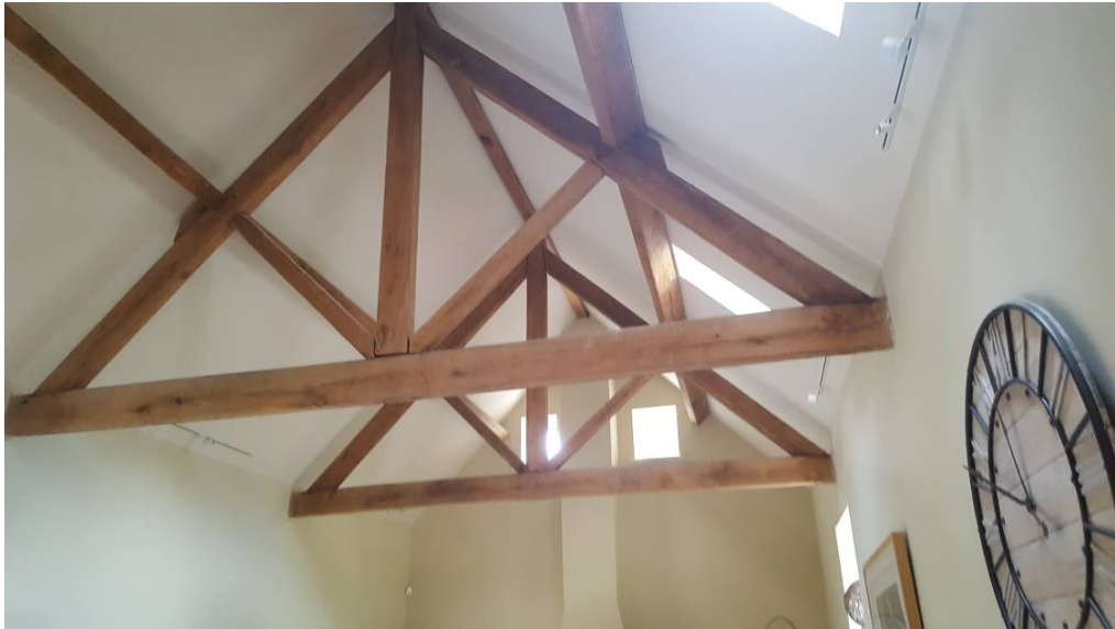
Exposed king post trusses and purlins to Sitting Room
