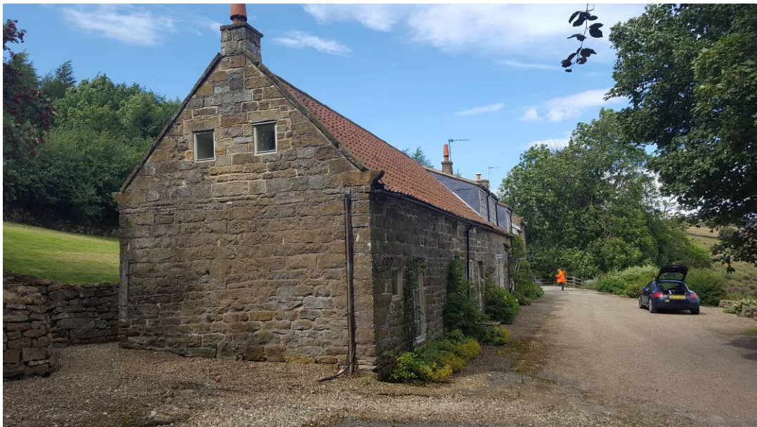
View of Existing Farmhouse Looking North West
