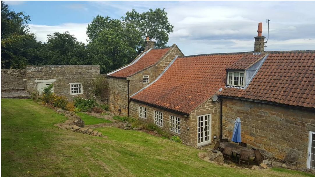
View of Existing Farmhouse Looking North West
