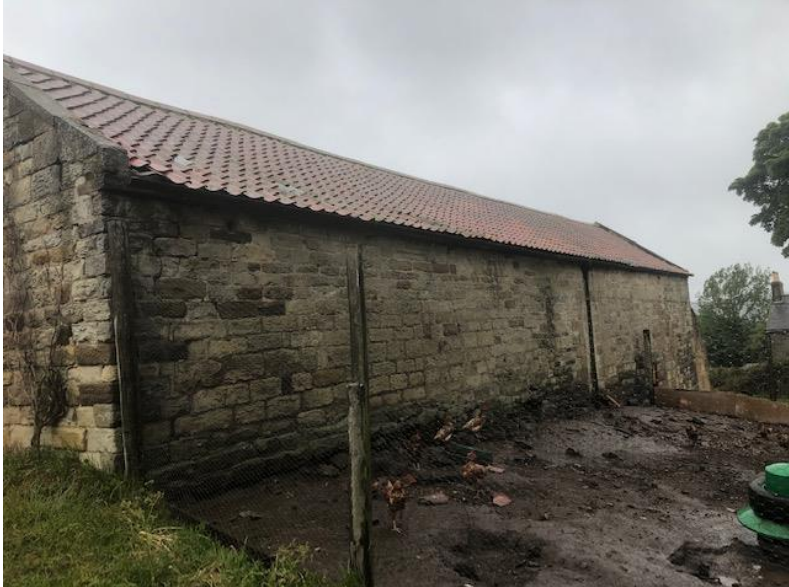
Photograph 8. Showing the north eastern elevation inside the chicken coup.
