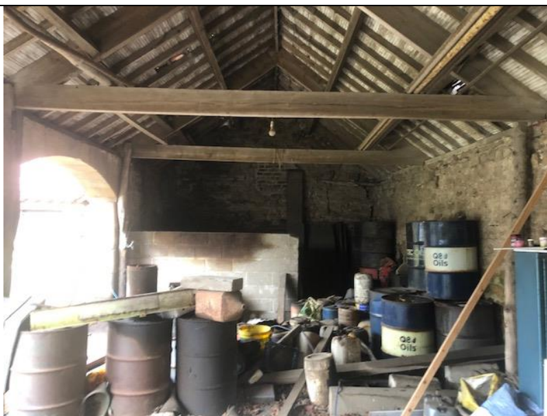
Photograph 19. Showing the storage area.
