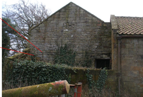
Photograph A north-east gable to eastern leg.
