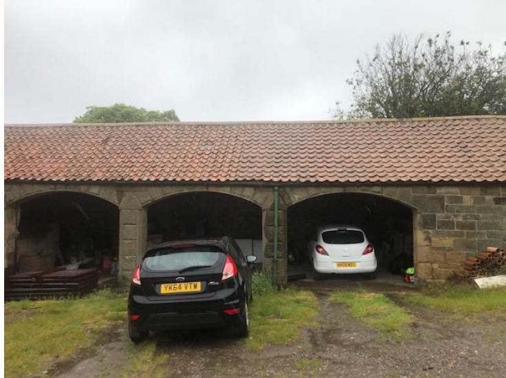
Photograph 2. Showing the external view of the south western elevation used for storage.
