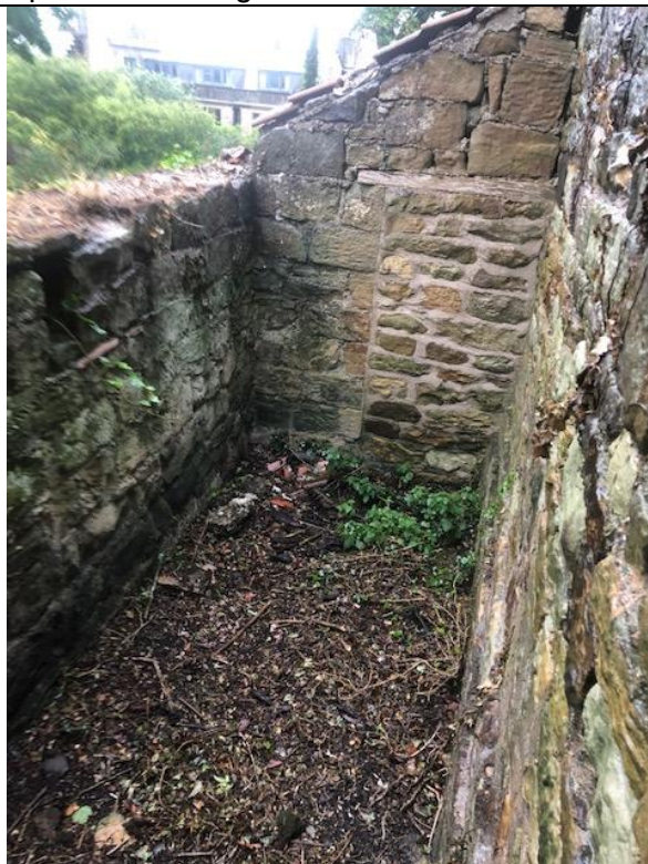
Photograph 30. Showing the internal view of the lean too with no roof
