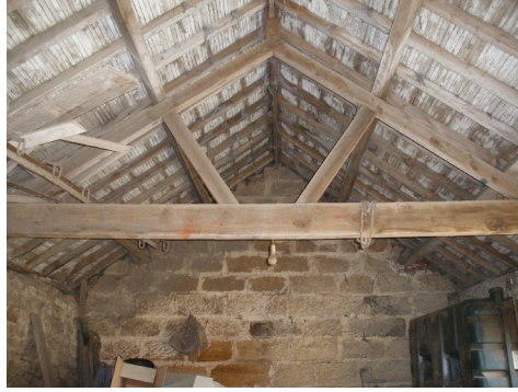
Photograph D roof truss and purlins arrangement
