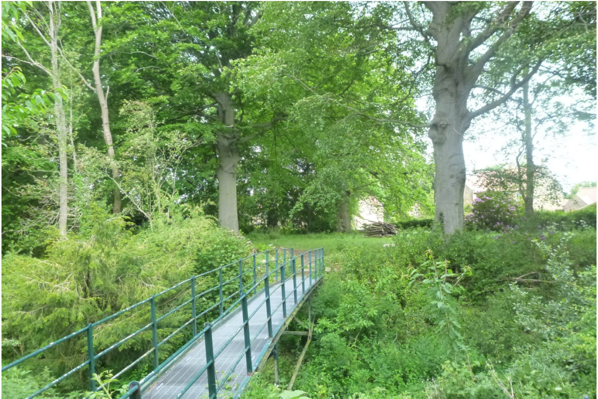
Existing bridge to be replaced with a new timber bridge.
