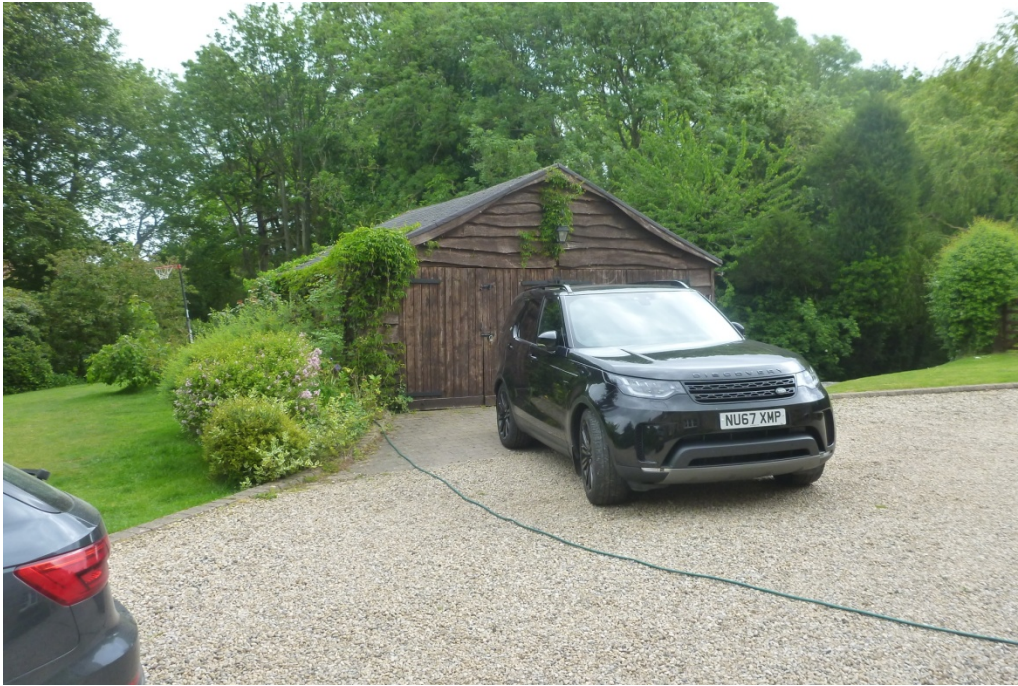
Existing garage to be replaced
