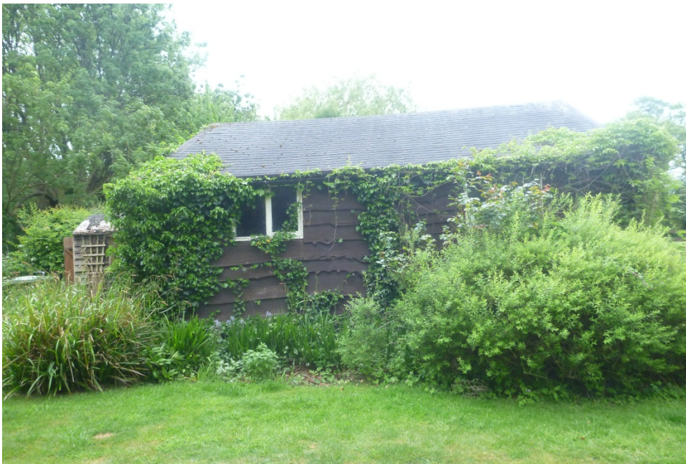
Existing garage building to be replaced
