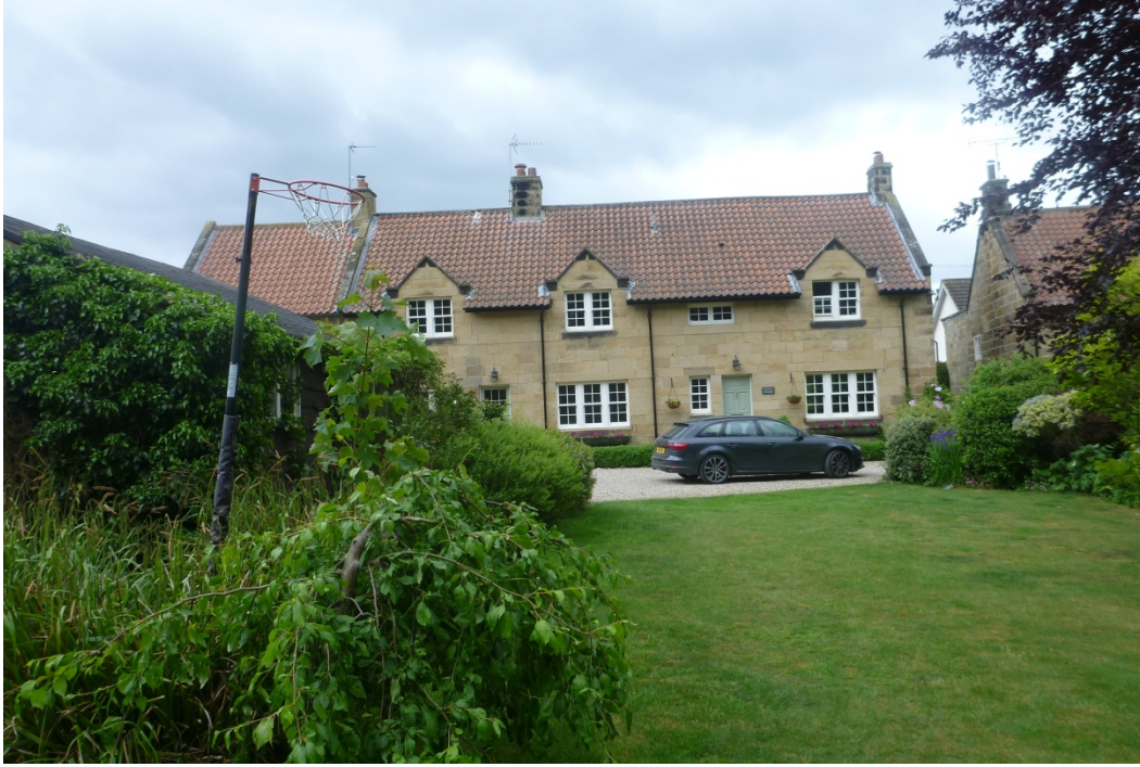
Front elevation viewed from the garden
