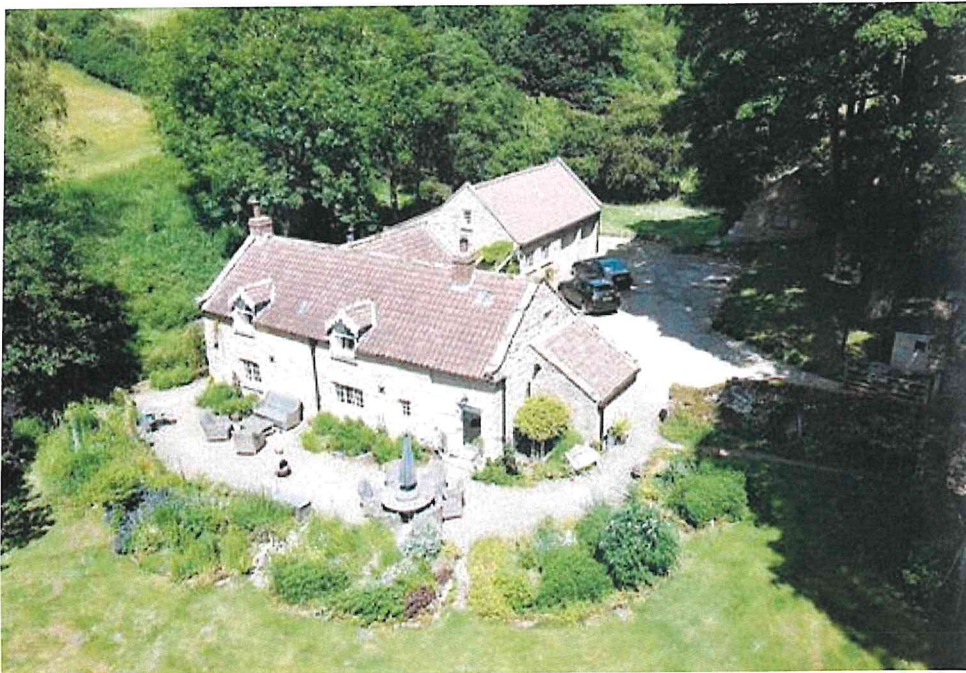
View of Lowdales Cottage from the South. The Southern range of the building is the original C17 cottage which would have had the roof lifted in the mid 19C by 800mm or so to give more generous attic accommodation and create the dormer windows. No work is proposed to this section of the house.
