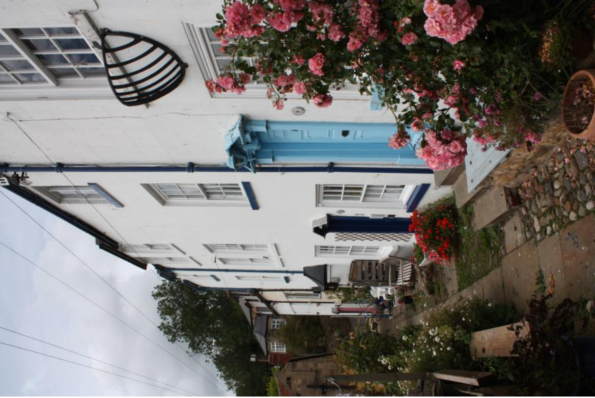
Photo 9: View west along Bloomswell with corner of No. 8 in foreground on RHS
