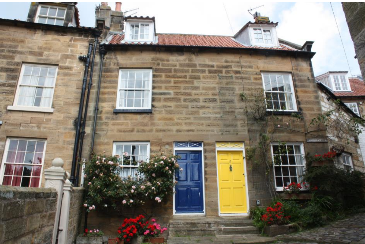
Photo 29: Brightly coloured doors to Grade II listed 4 & 5 Sunny Place (within the conservation area)
