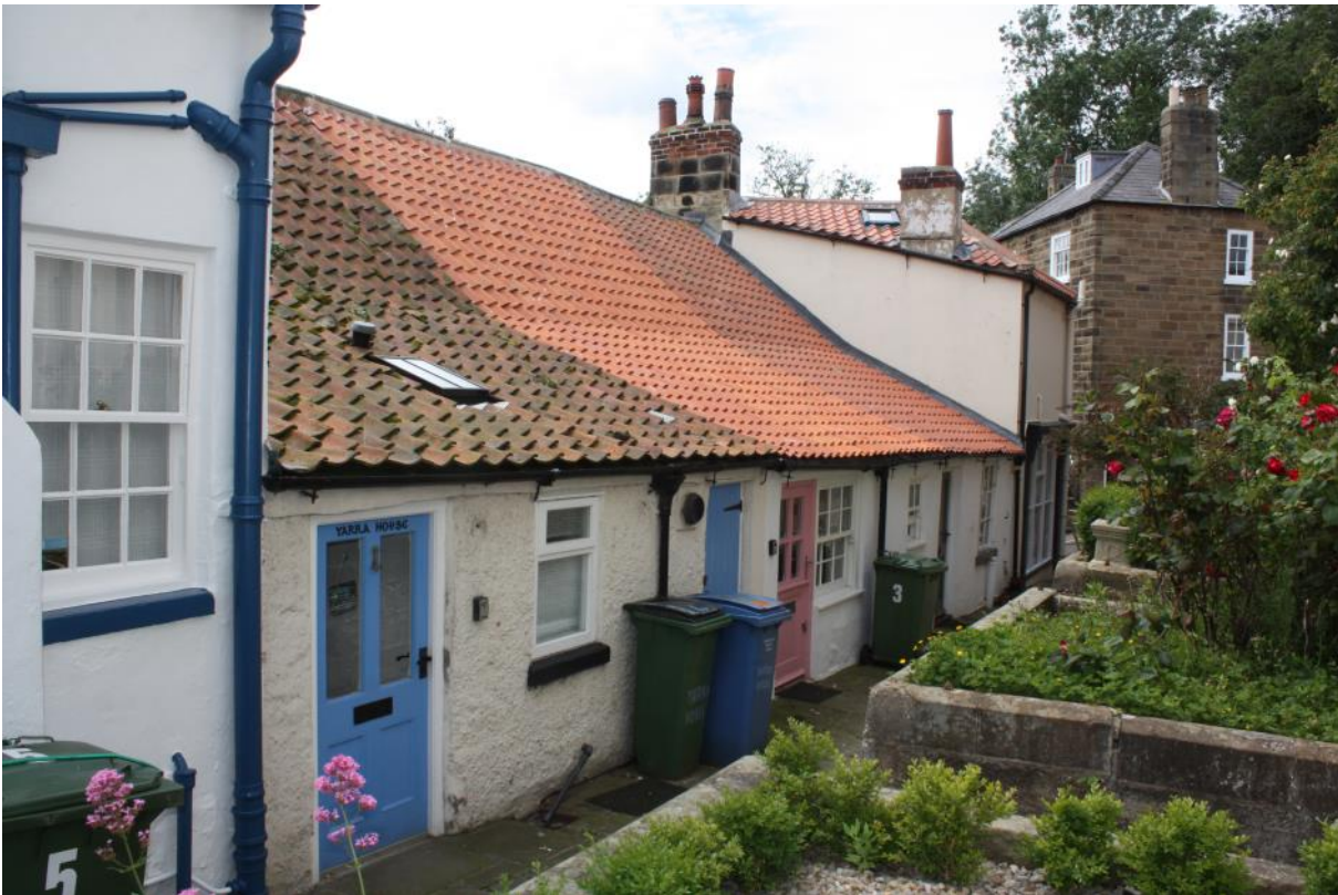
Photo 3: View of north elevations of Nos. 1-4 Bloomswell, looking west along the back lane
