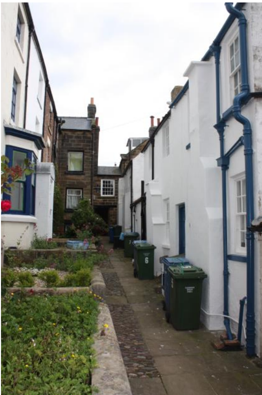
Photo 4: View of north elevations of Nos. 5-9 Bloomswell, looking east along the back lane
