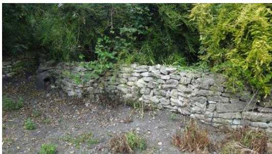
Photograph 19. North Side towards North West Corner
