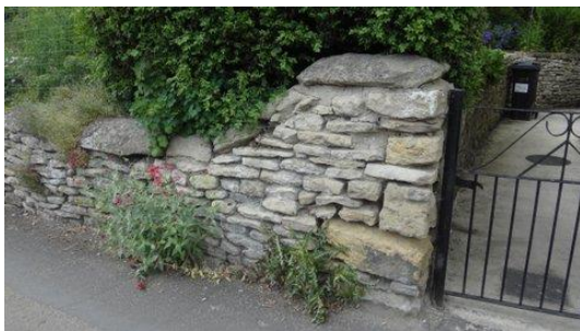
Photograph 15. Position J (External Wall)
