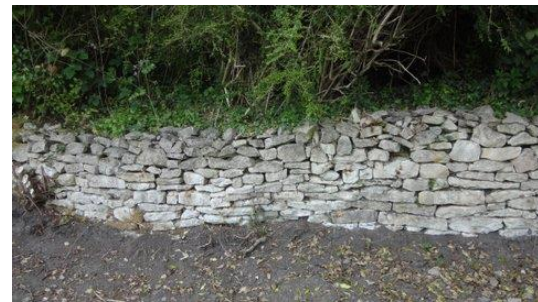
Photograph 22. West Side adjoining Brookfield
