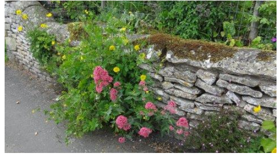
Photograph 14. Position H (External Wall)
