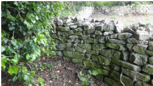
Photograph 5. Position C (External Rebuilt Wall – Former Gate Position)
