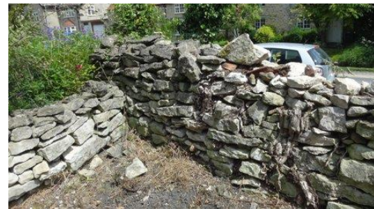
Photograph 8. Position D (Internal Wall)
