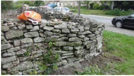
Photograph 1. Position A (External Wall)
