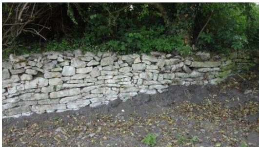
Photograph 21. West Side towards North West Corner
