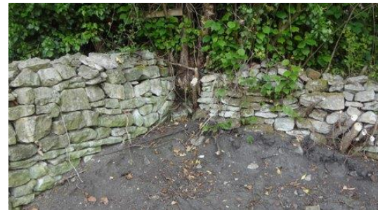
Photograph 6. Position C (Internal Rebuilt Wall – Former Gate Position)
