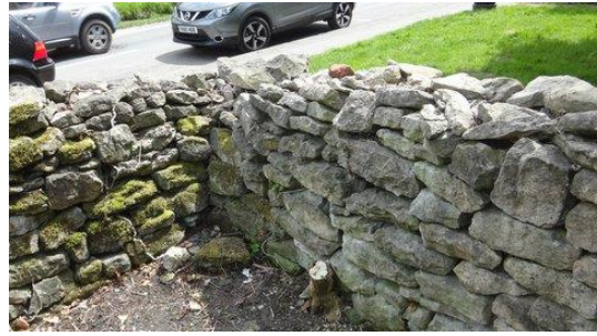
Photograph 2. Position A (Internal Wall)
