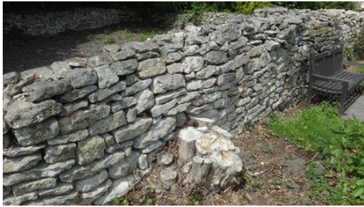
Photograph 11. Position F (External Wall)
