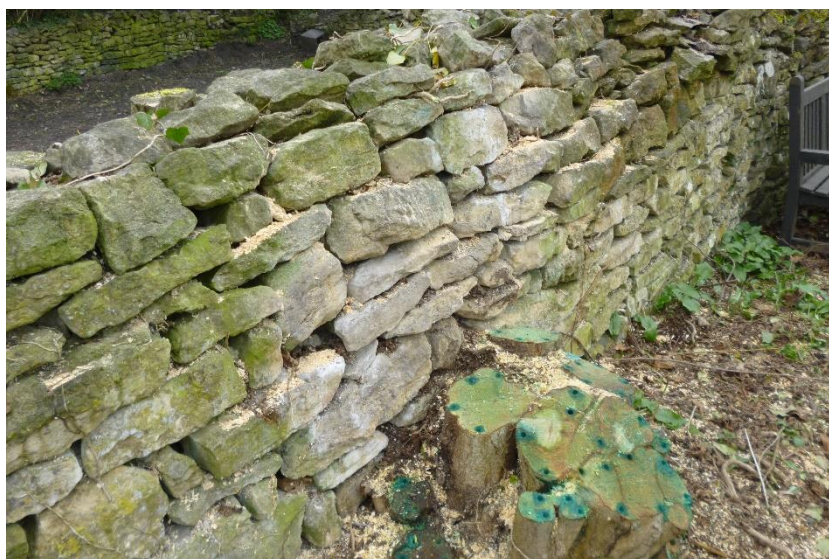
The treated stump of the Hazel Tree immediately following removal (Photograph by Contractor)
