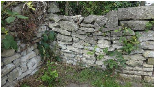
Photograph 7. Position D (External Wall)
