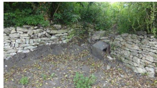
Photograph 20. North West Corner
