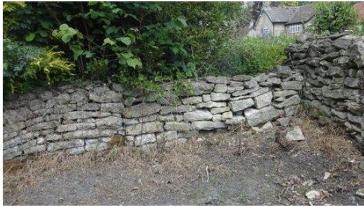
Photograph 17. North East Corner
