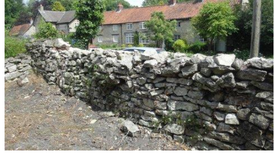
Photograph 10. Position E (Internal Wall)
