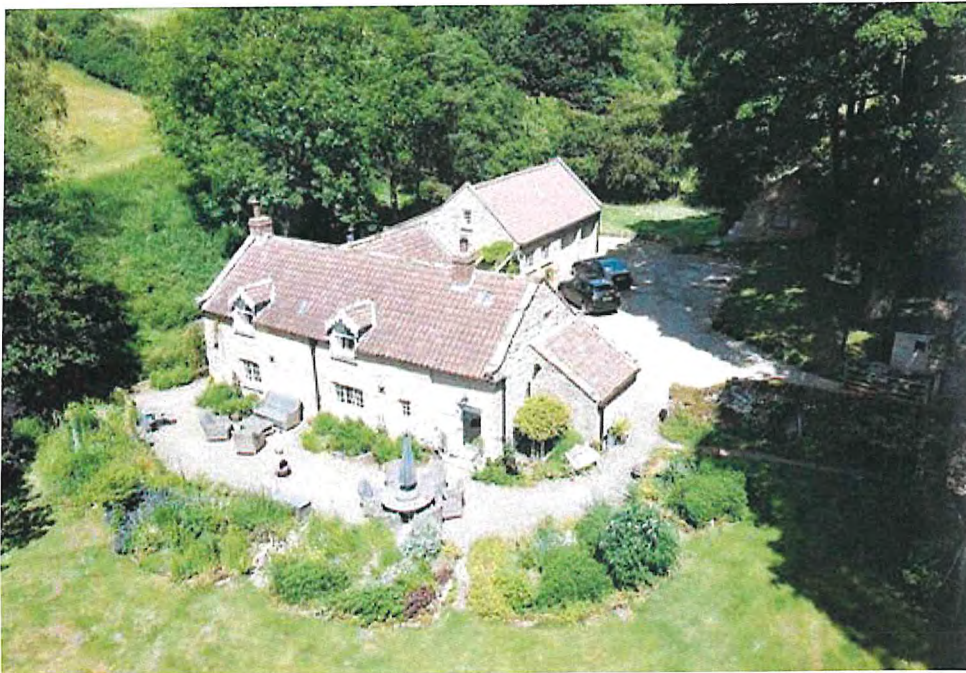
View of Lowdales Cottage from the South. The Southern range of the building is the original C17 cottage which would have had the roof lifted in the mid 19C by 800mm or so to give more generous attic accommodation and create the dormer windows. No work is proposed to this section of the house.
