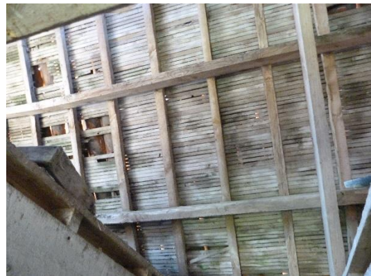
Photo 4 Wooden lath lining and wood floor
