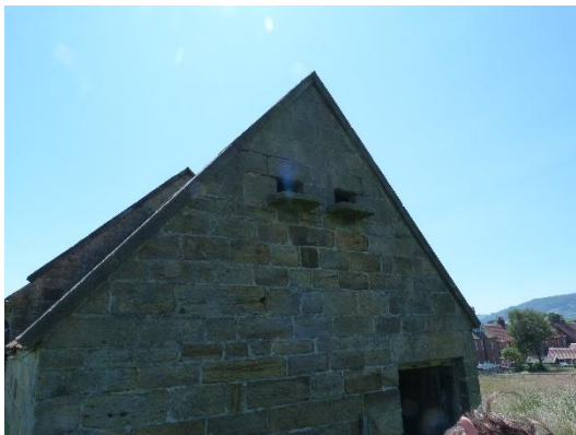
Photo 13 Access holes to dovecote
