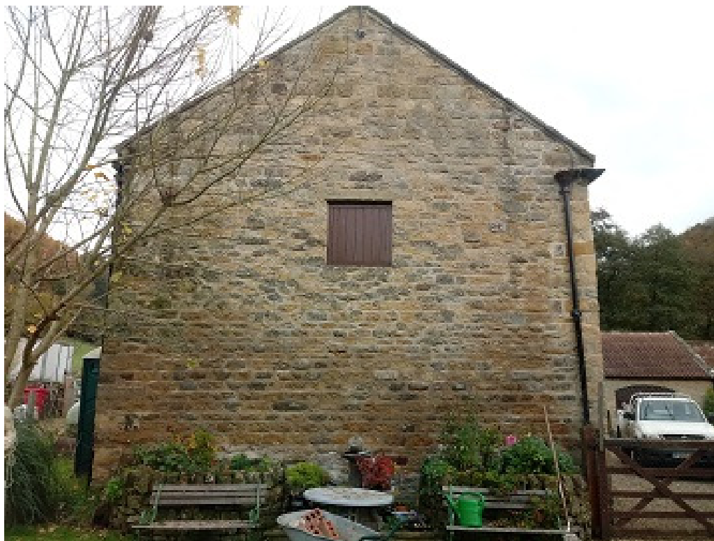
Plate 2. Looking towards the south gable
