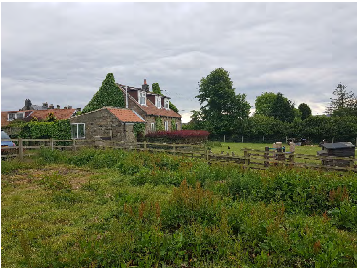
4. View of eastern part of site looking south with The Forge in the middle ground and Rowena cottage in the back ground.
