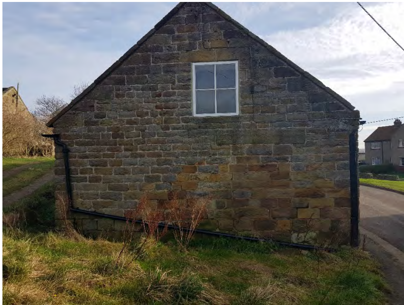
5.25 View of western gable end: Looking east.
