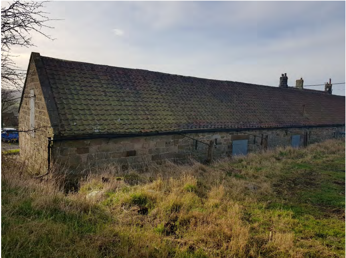
5. View of outbuilding from proposed rear courtyard garden area looking southwest
