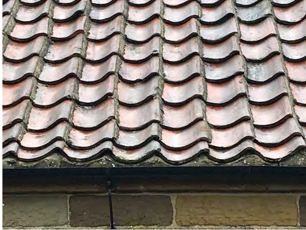
Clay pan tile roof covering
