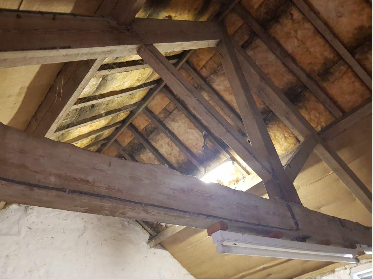
7. View of interior roof rafters
