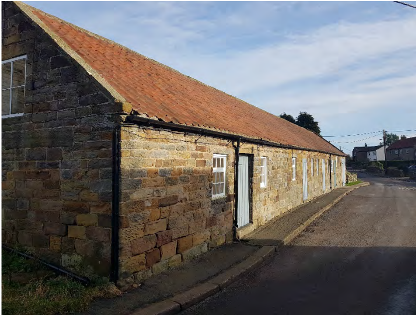
5.23 View of outbuilding frontage: Looking east.
