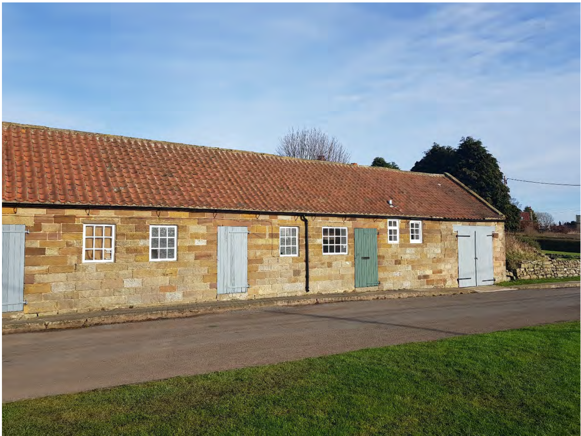
2. View of the building looking north from lower fork of road
