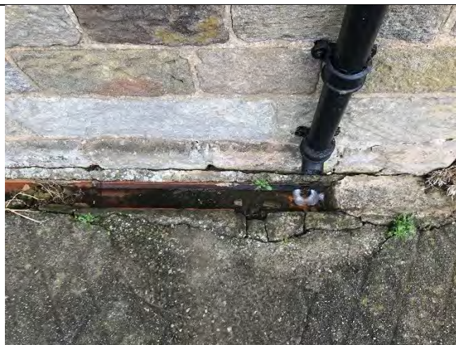
Cast Iron rainwater goods to village combined drain.
