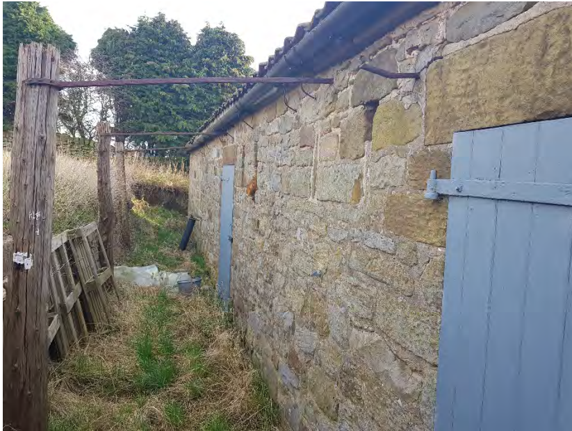
5.27 View of rear of outbuilding: Looking East.
