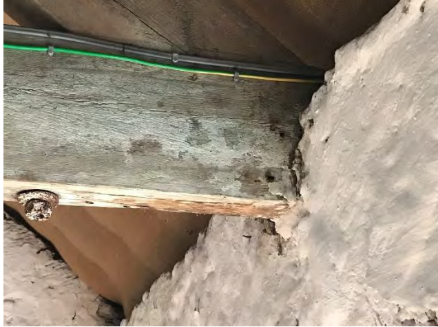
King Post Truss foot.
