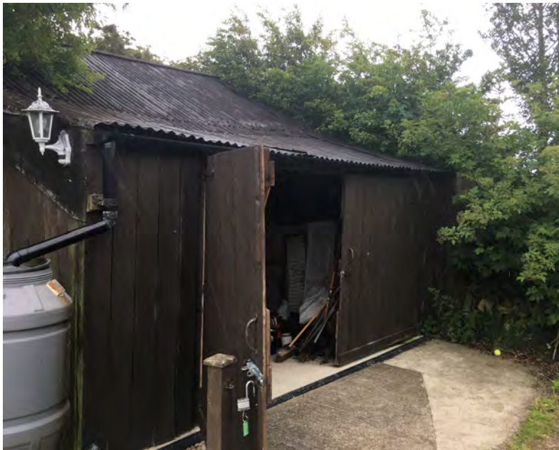
Fig. 3: View of existing building.
