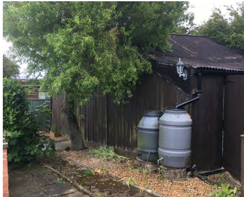
Fig. 4: View of existing building.
