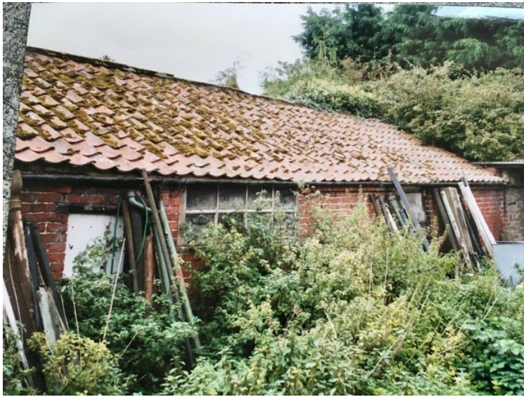
One of the previously existing buildings within / abutting the application site.
