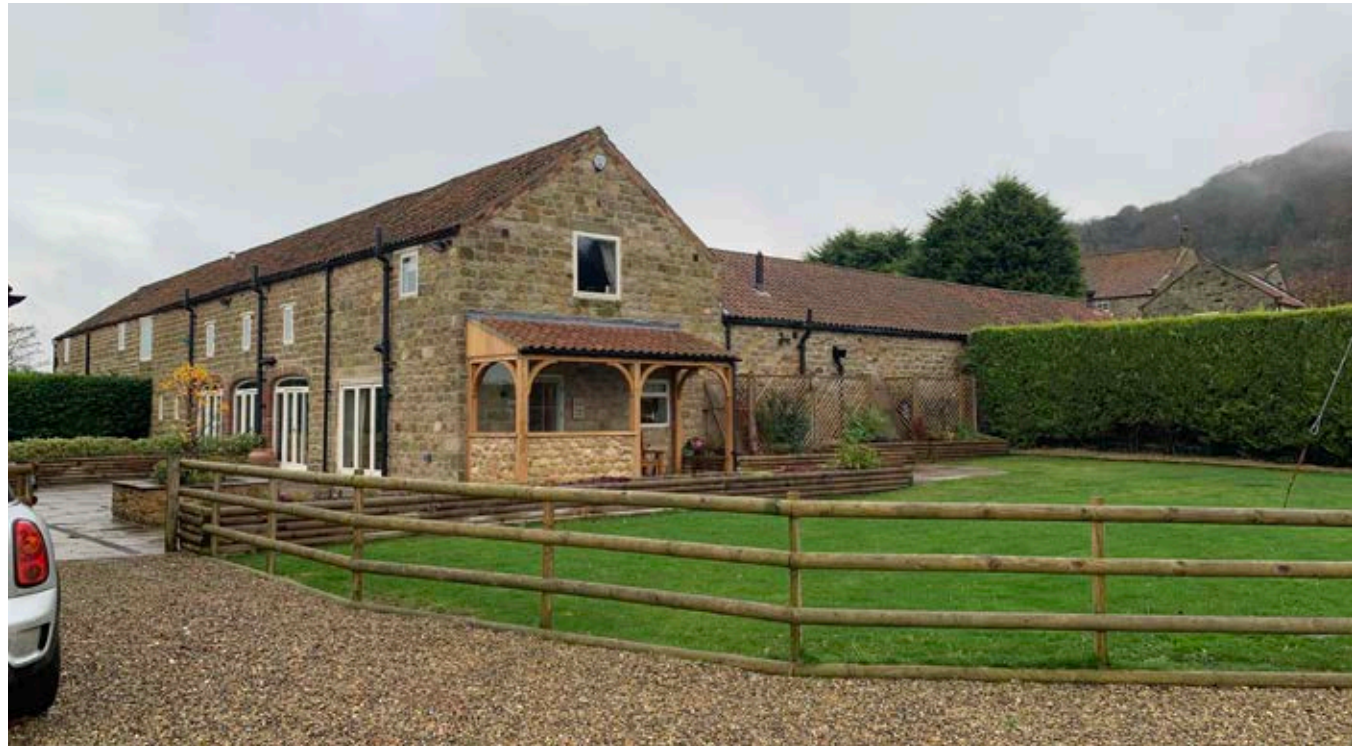
Arrival and north east side of barn
