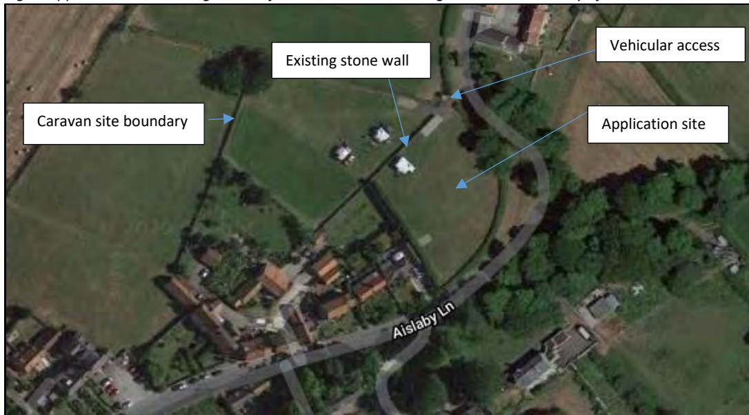
Fig 1: application site showing extent of caravan site and existing stone wall boundary of site
