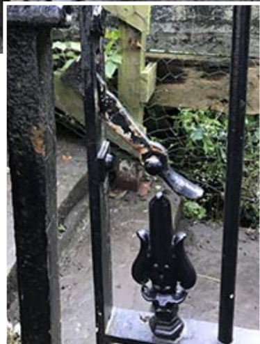
detail of existing gate
