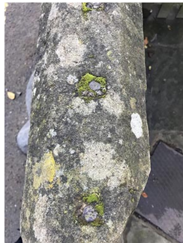
detail of top of stone wall where the railings were removed
