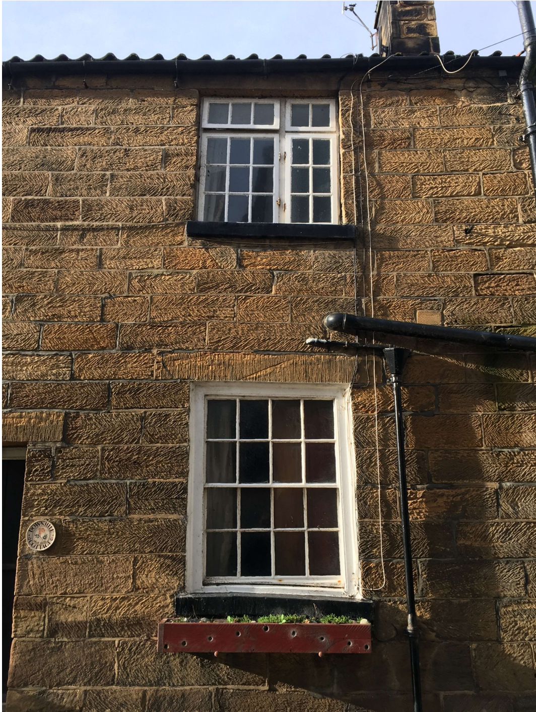
Photograph 1 W4, First floor window
