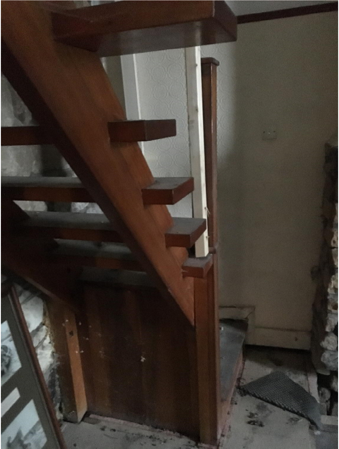
Photograph 1 Open plan stair to lounge
