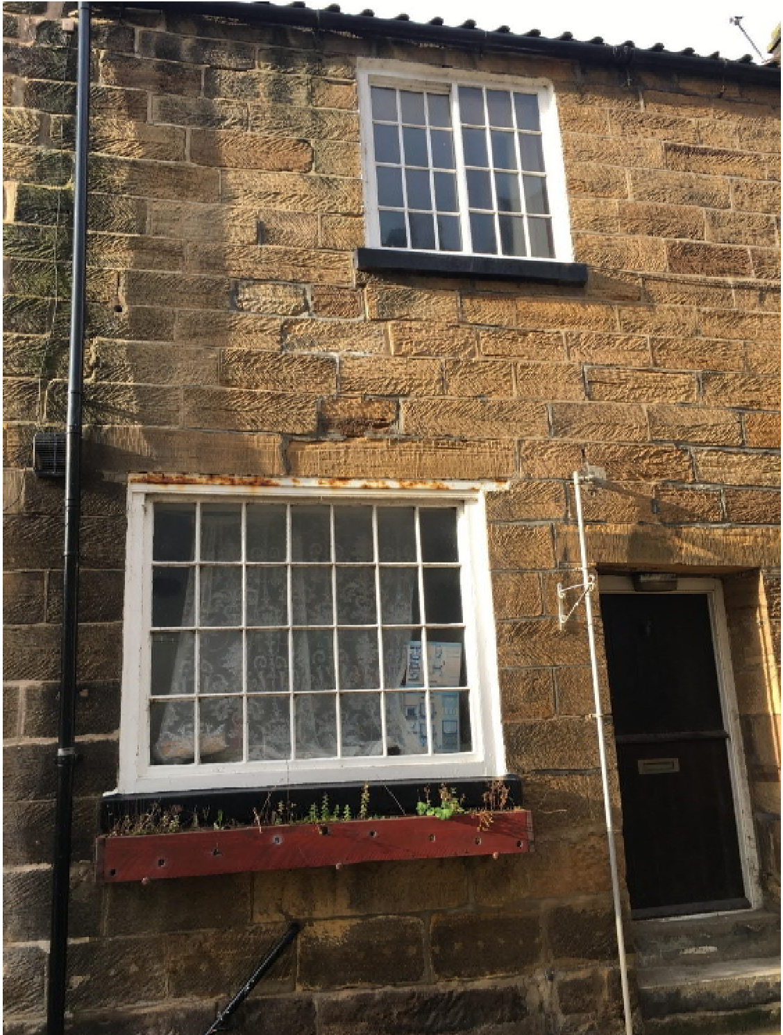
Photograph 5 Part Front Elevation, W1 and W3
