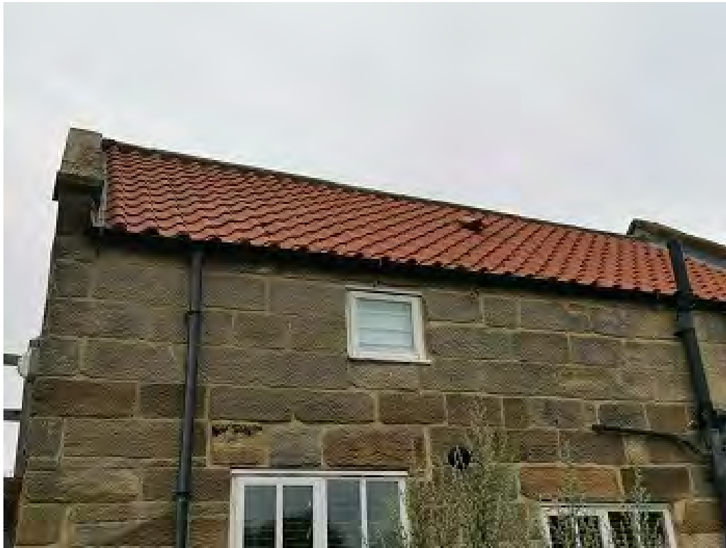
Plate 8. Shows east elevation of Building 3
