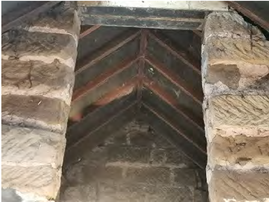
Plate 3. Shows timber roof supports and opening between rooms.
