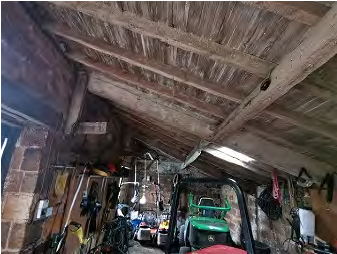
Plate 5. Shows internal roof supports and lining in Building 2.
