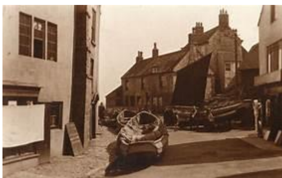
Fig 5. New Road, Close to Albion Street, Robin Hoods Bay –
