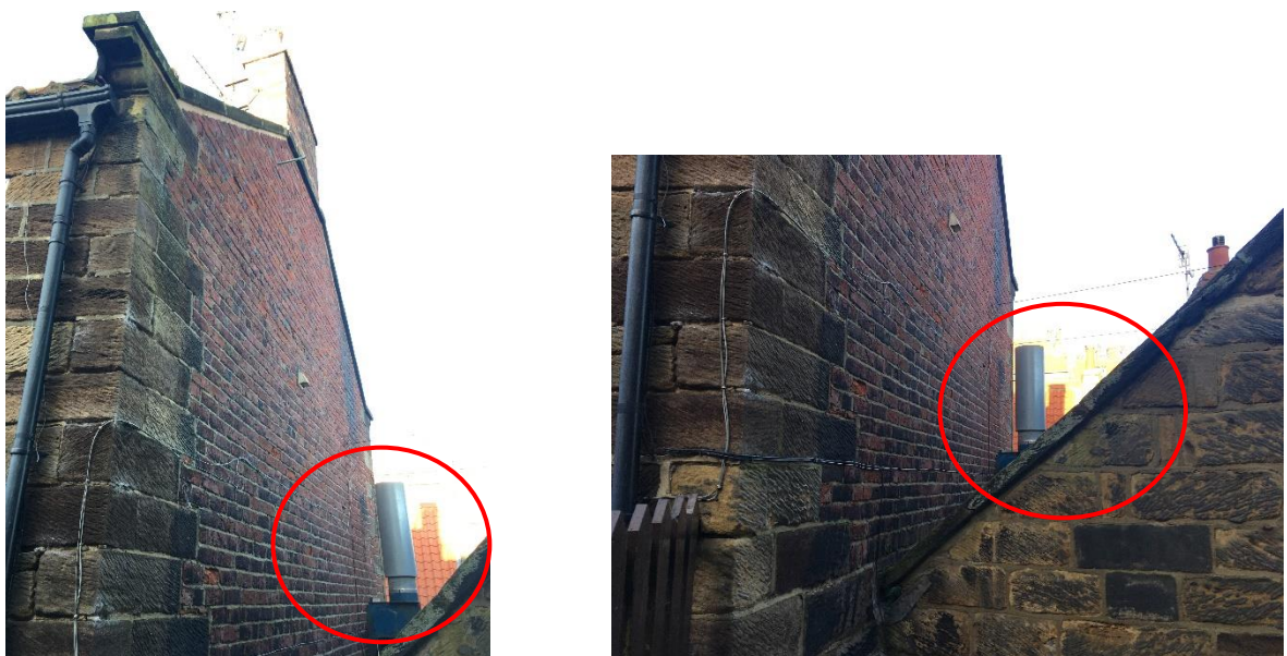
Fig 6 & 7. – Existing steel flue existing between Maryondale and overhanging neighbouring property.
