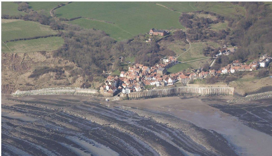
Photo 1 Aerial picture showing the Sea Wall
