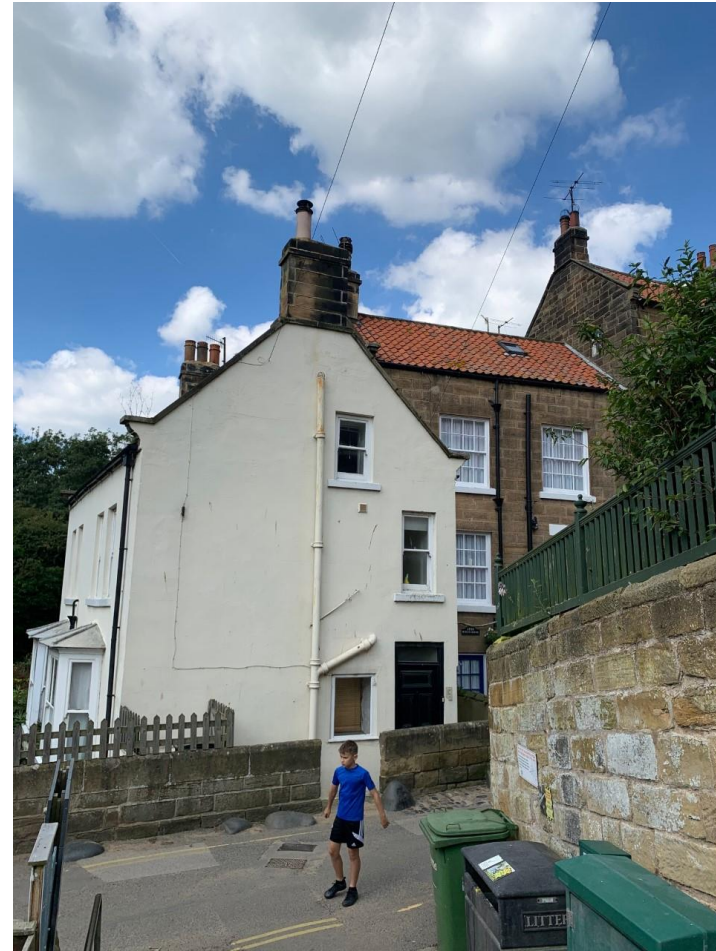
Image 6 – Current view of the properties New Road Elevation taken from the bridge in August 2020.
