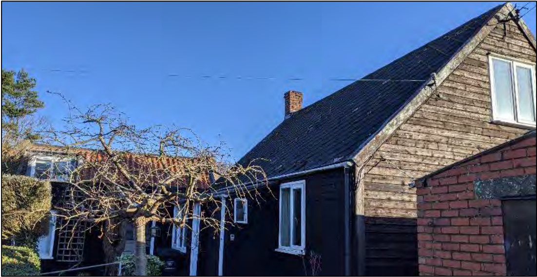
Plate 4. Room within roof of B1
