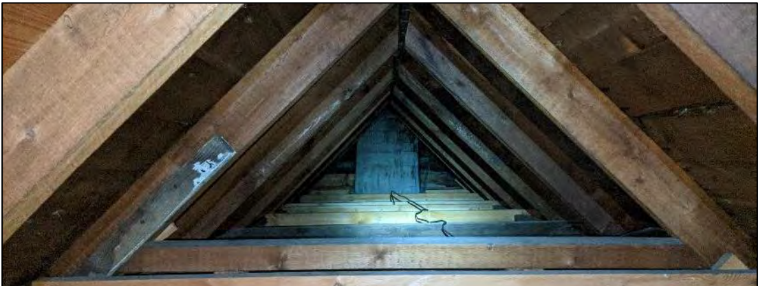
Plate 5. Small void (0.5m high) present in B1
