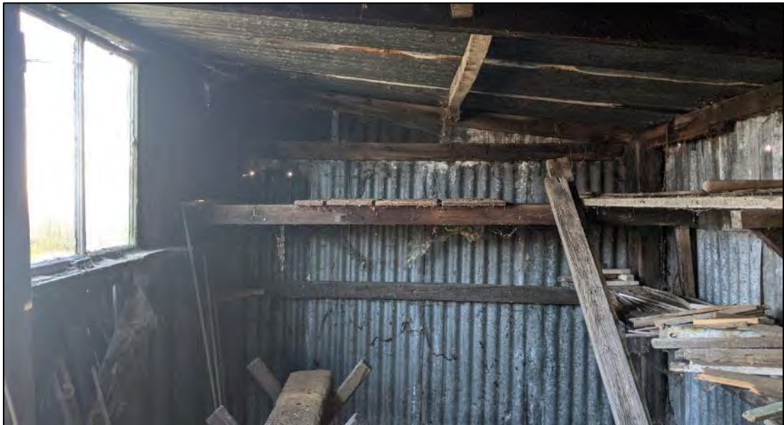
Plate 12. Interior of B5
