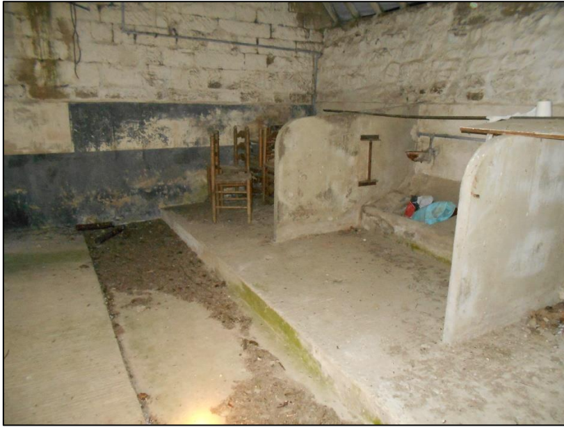
Figure 11: Interior of western side of barn
