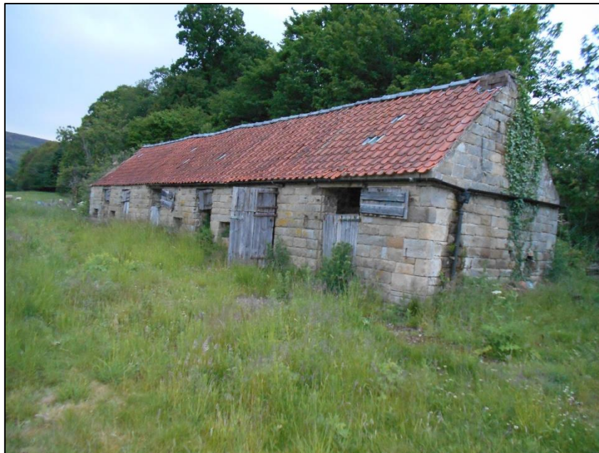
Figure 15: South side of building
