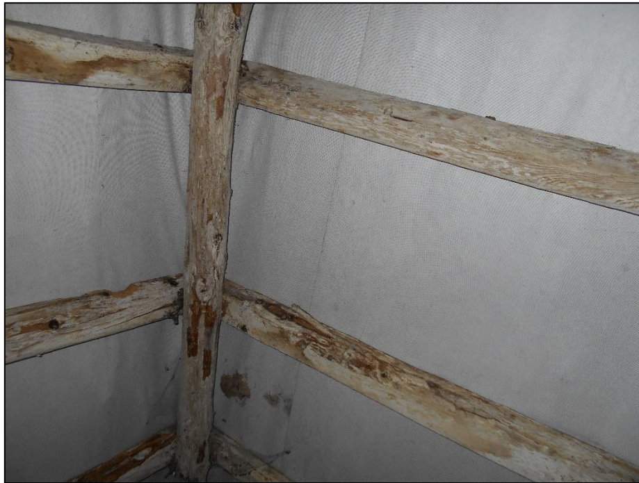
Figure 6: Underside of roof
