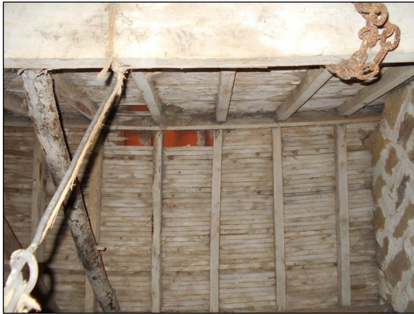
Figure 16: Underside of roof
