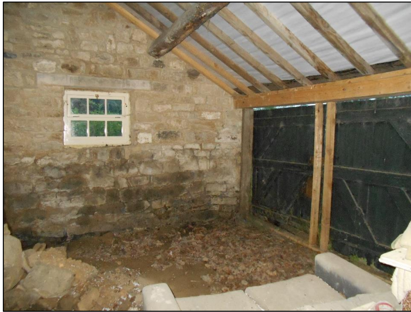
13: Interior of part of eastern single storey section beneath catslide roof
