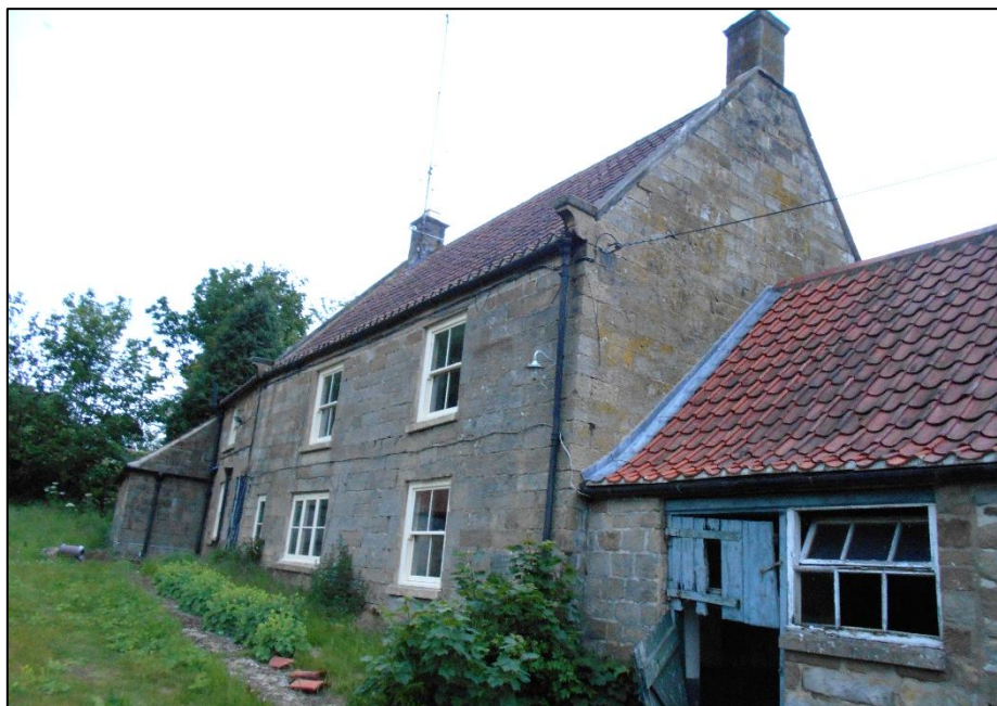
Figure 4: West side of the house
