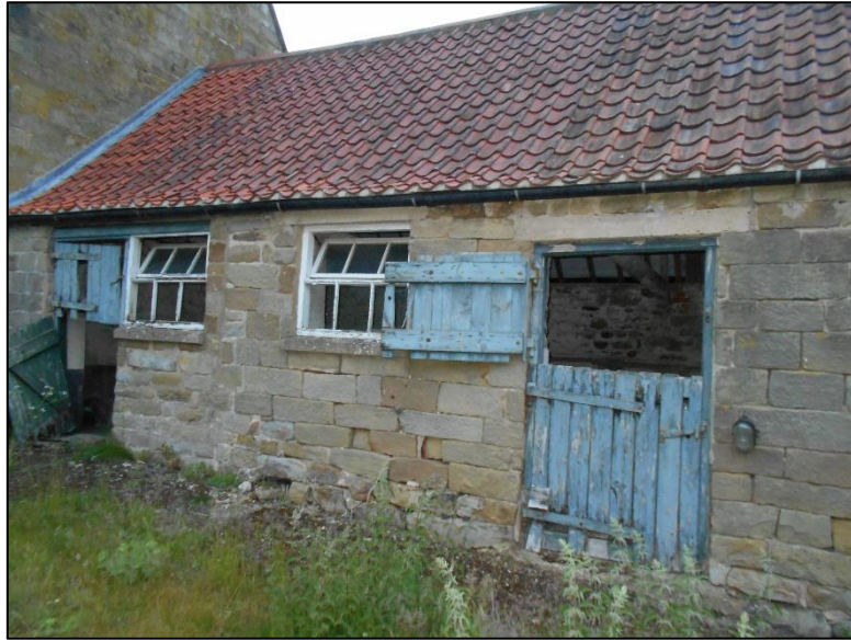
Figure 7: Northern end of barn, west side
