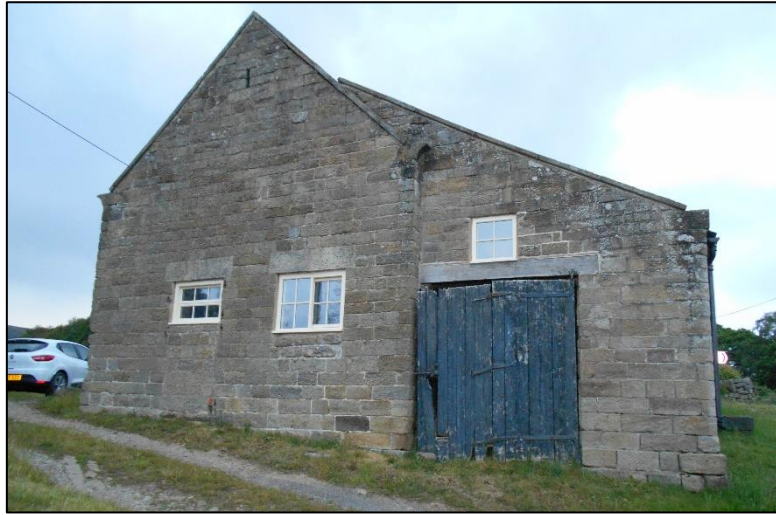
Figure 9: South end of barn
