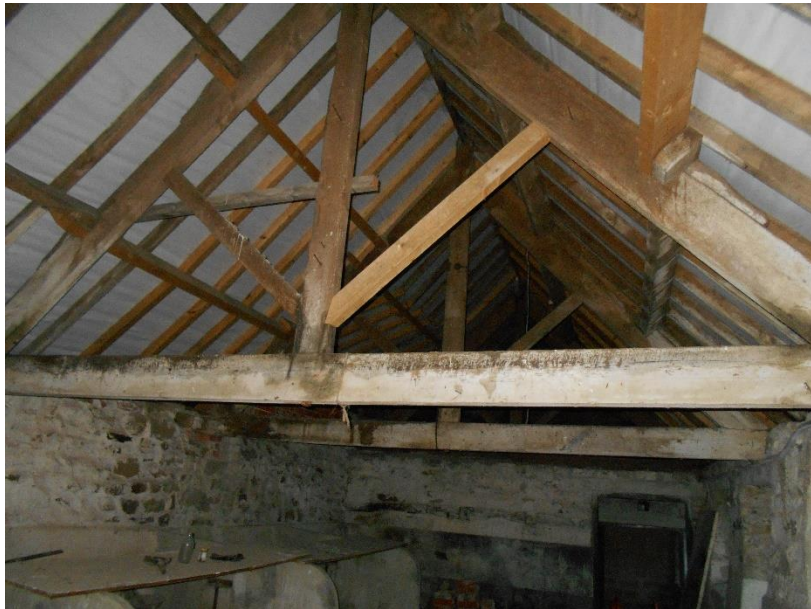
Figure 12: Underside of roof, south end of building
