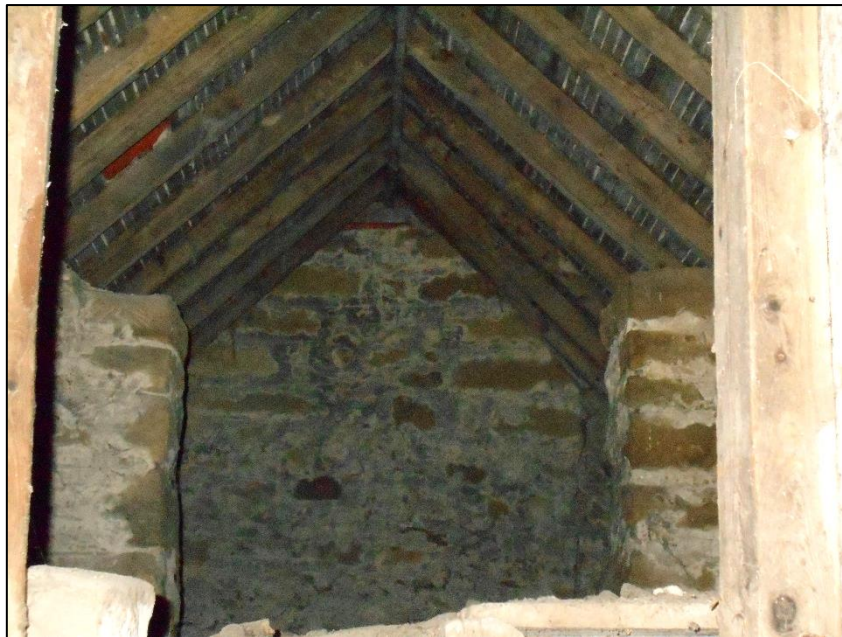
Figure 17: View westwards through roof void
