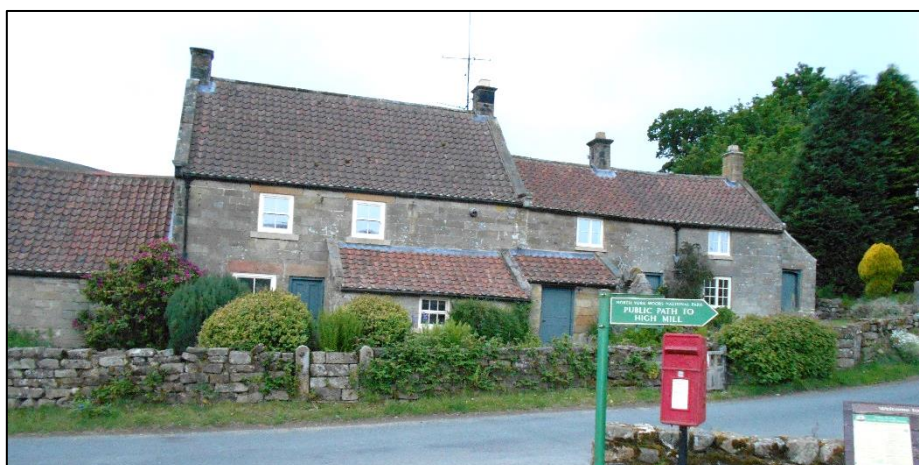
Figure 5: East side of the house
