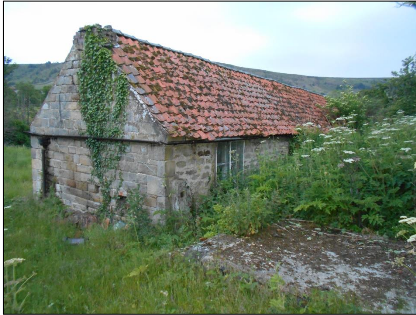
Figure 14: North side of building
