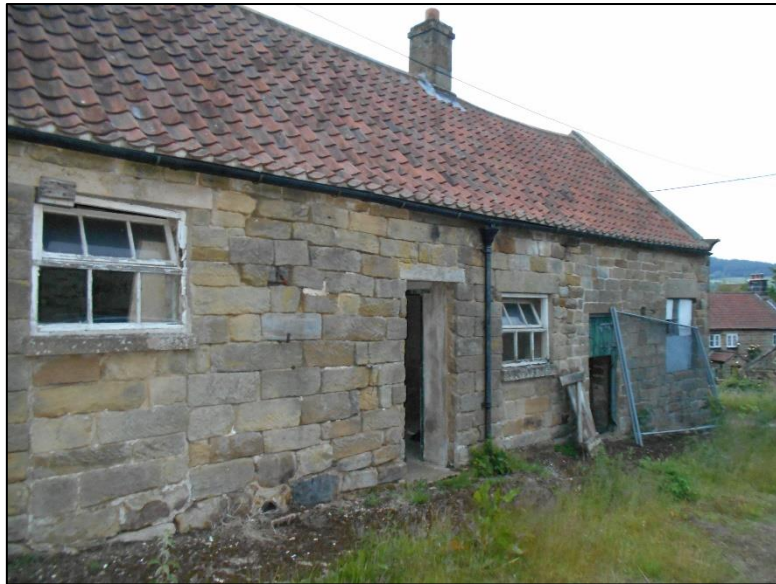
Figure 8: Southern end of barn, west side
