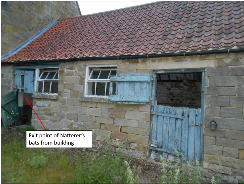
Figure 19: Emergence / access point of Natterer's bats from building
