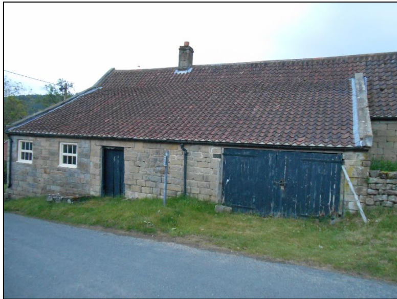
Figure 10: Southern end, east side showing cat-slide roof
