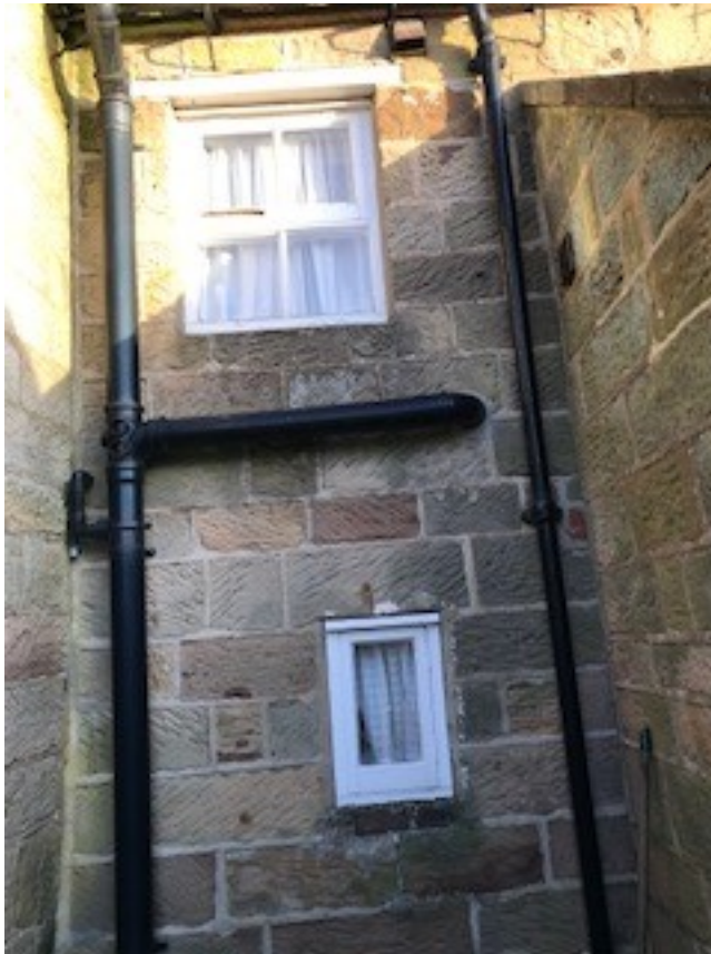
CLOAKROOM WINDOW (ground floor) and BATHROOM WINDOW (first floor)
