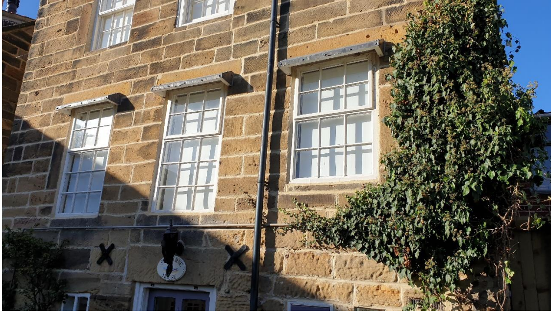
Image 5: first floor windows
