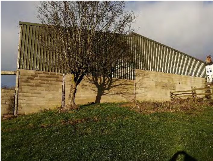
Photo 5 – building 1. South elevation following work.
