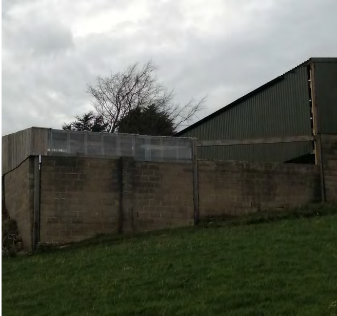
Photos 12 – building 3. Current view southern elevation showing existing concrete block wall.
