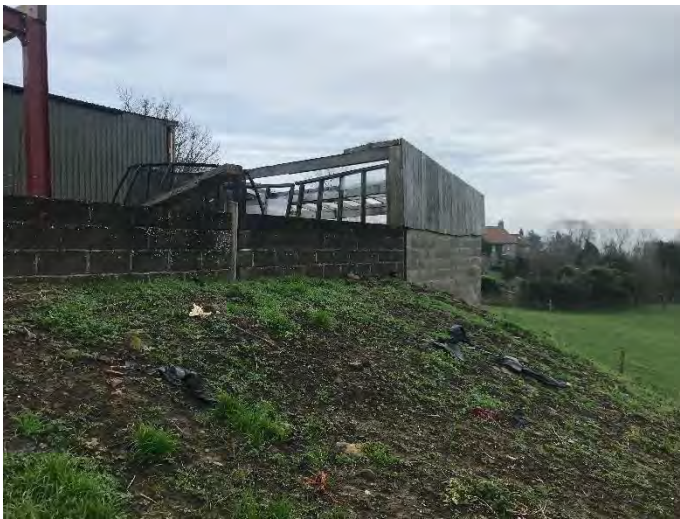
Photo 11 – building 3. Current view north west elevation.
