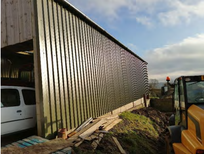
Photo 4 – building 1. West elevation following work.
