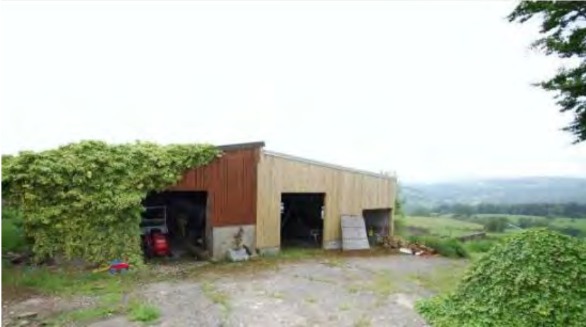
Photo 1 – building 1. Northern elevation prior to work.
