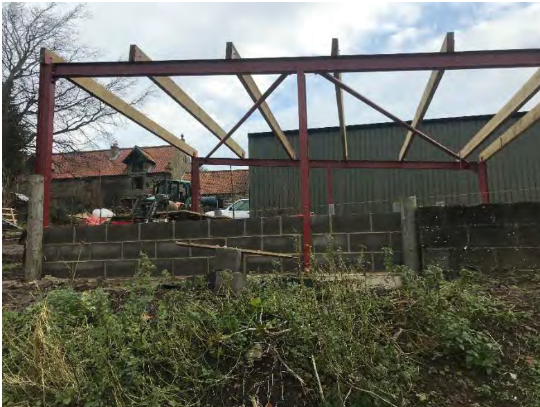
Photo 9- building 2, west elevation. Part constructed.
