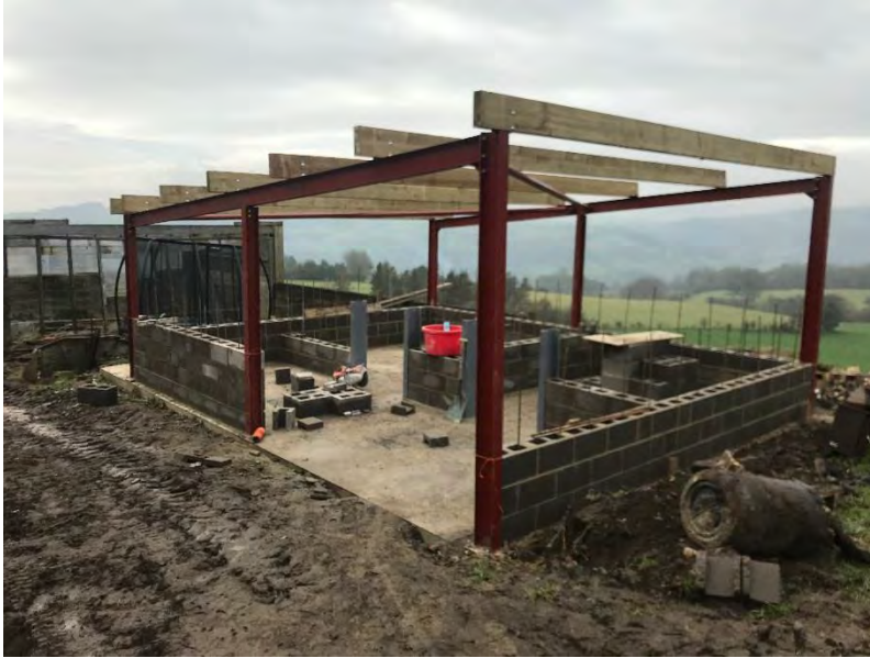
Photo 8 – building 2, north east elevation. Part constructed.
