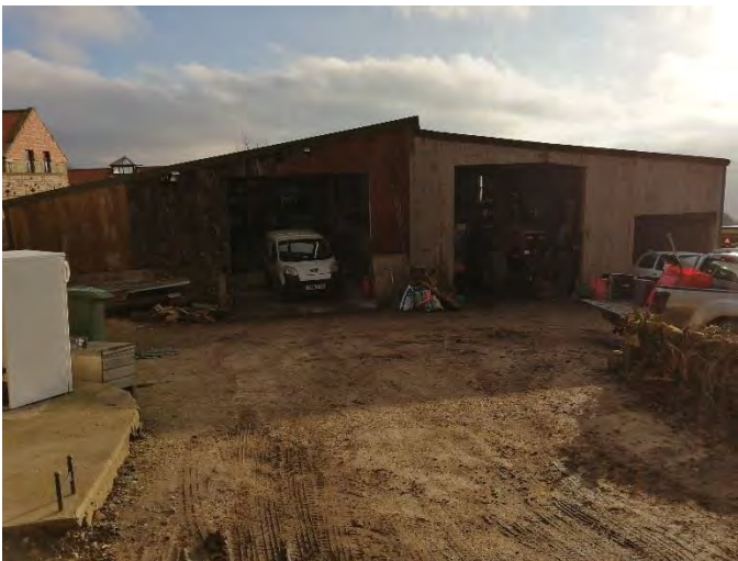
Photo 3 – building 1. North elevation following work to enlarge access.
