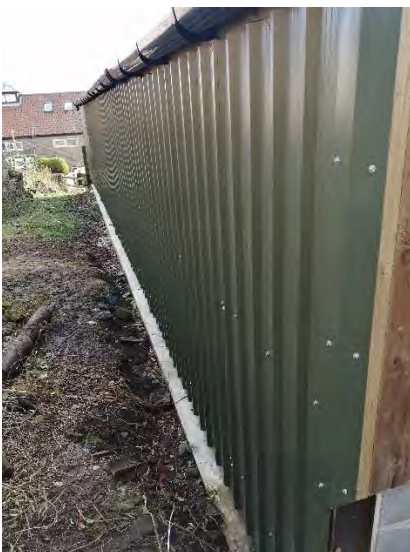
Photo 6 – building 1. East elevation following work.
